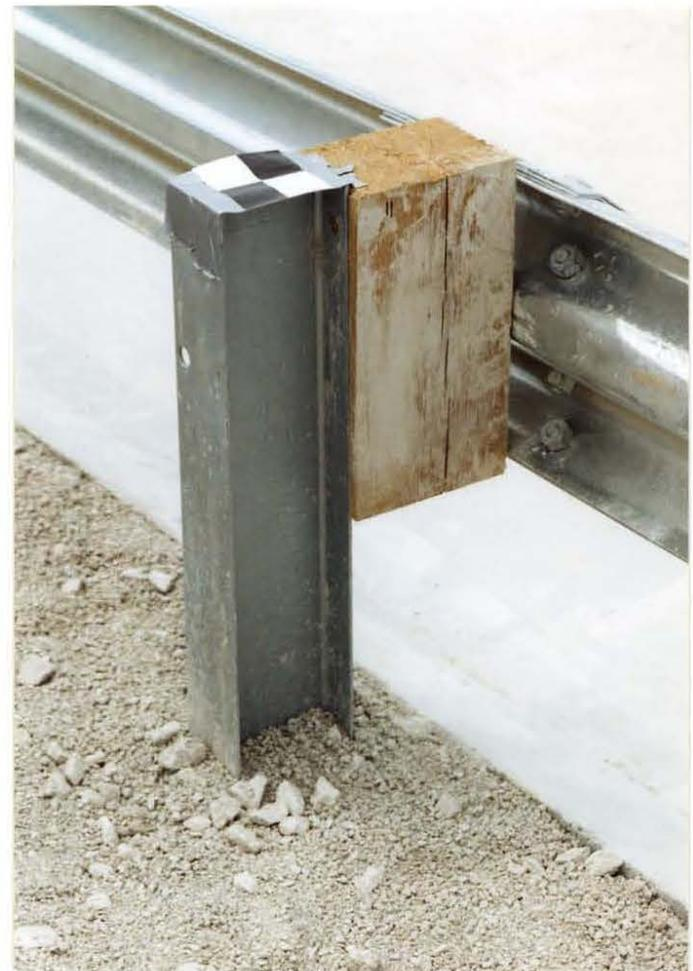
Figure 3. Post-to-Rail Attachment for the Guardrail Over Curb System
