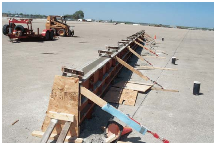
Figure 10. Permanent New Jersey Safety Shape Barrier System Construction
