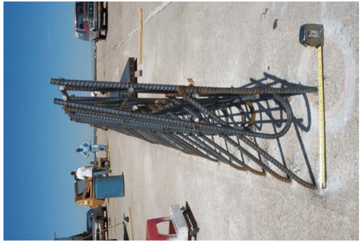
Figure 9. Permanent New Jersey Safety Shape Barrier System Reinforcement
