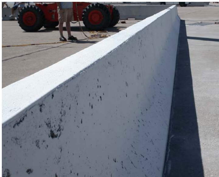
Figure 11. Permanent New Jersey Safety Shape Barrier System
