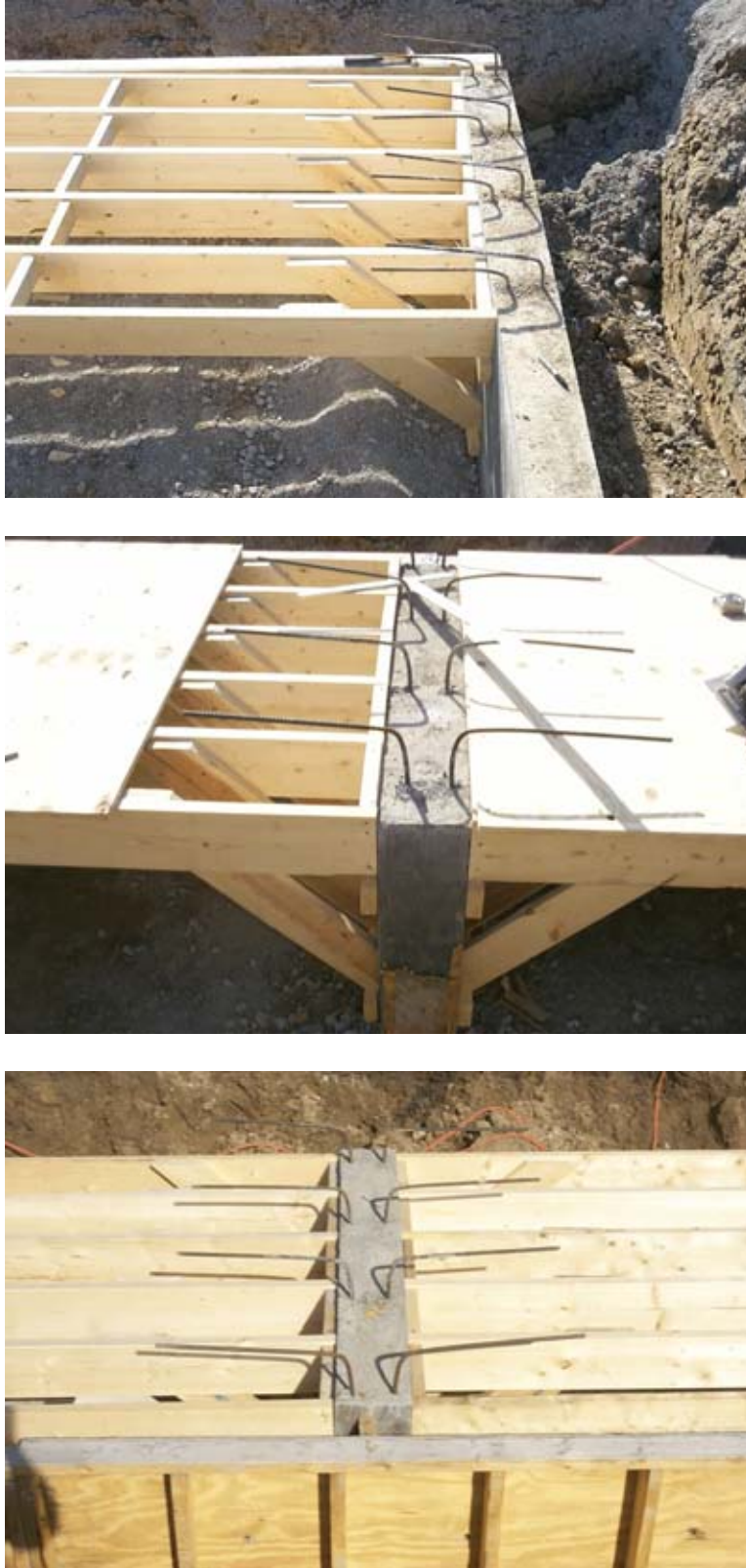
Figure 18. Concrete Culvert Walls and Top Slab Formwork
