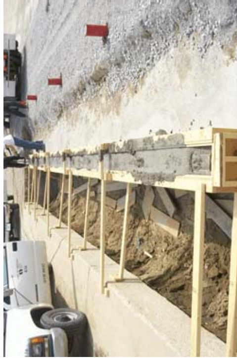
Figure 20. Concrete Culvert Curb Construction
