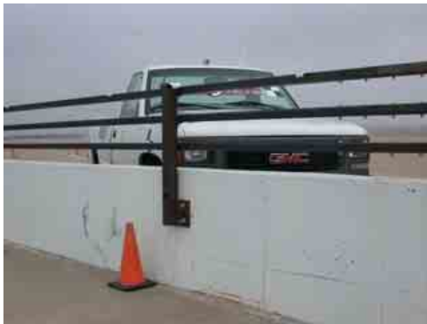
Figure 8. Combination Traffic/Bicycle Bridge Rail
