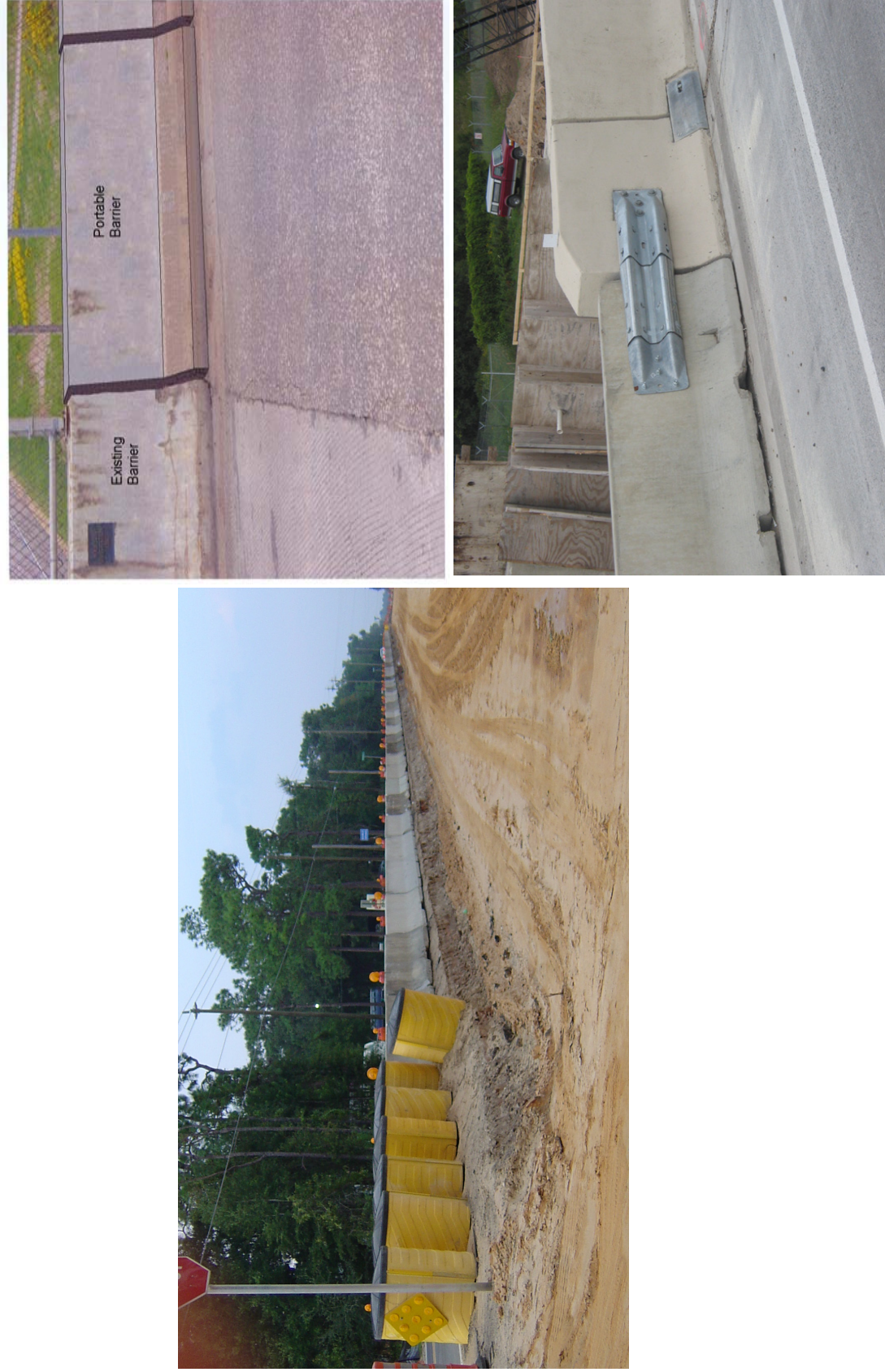
Figure 1. Temporary Concrete Barrier Installations on Asphalt: a) Near Drop-Off and b) Transition to Rigid Barrier
