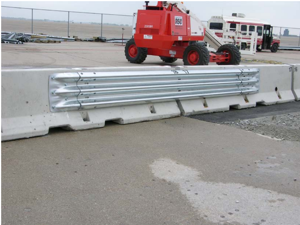
Figure 46. Free-Standing to Rigid Concrete Barrier Transition Photographs
