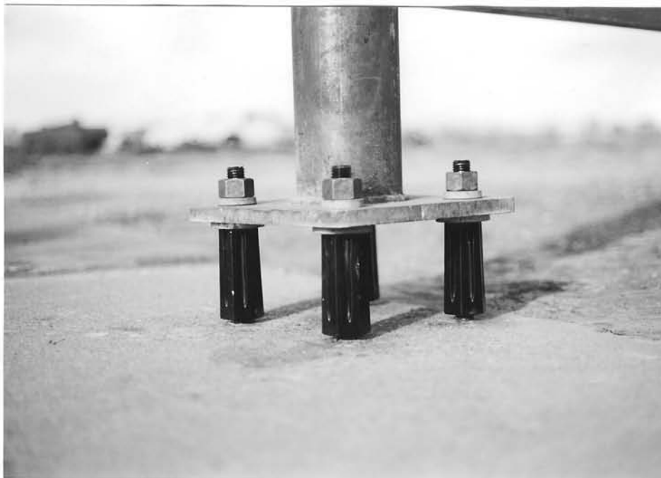
Figure 10. Installed Breakaway Couplings
