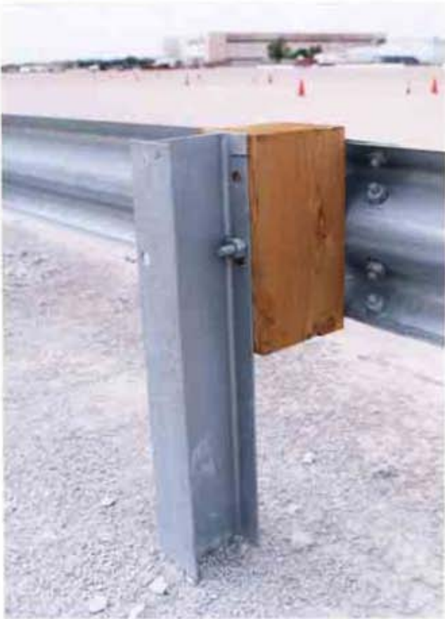
Figure 4. Post-to-Rail Attachment for the Type B (W-beam) Longitudinal Barrier System
