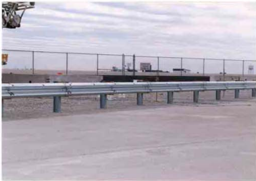
Figure 2. Modified Type B (W-beam) Longitudinal Barrier System
