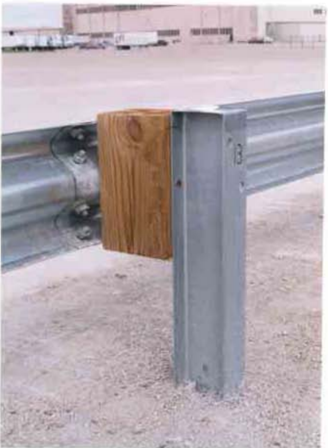
Figure 4. Post-to-Rail Attachment for the Type B (W-beam) Longitudinal Barrier System
