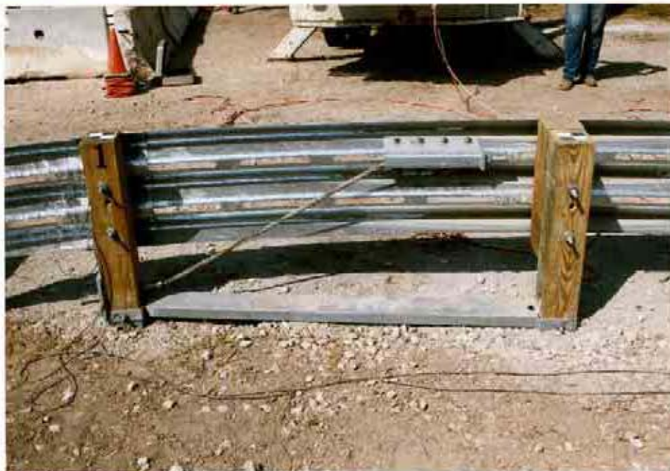
Figure 12. Bullnose Barrier Design
