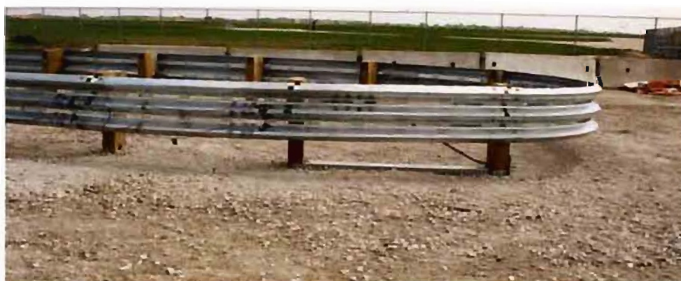
Figure 8. Bullnose Barrier Design
