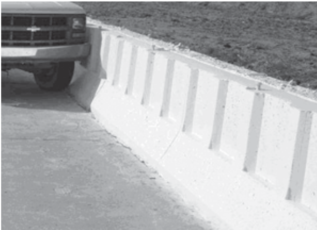
Figure 38. Examples of Texturing [38] and Vertical Asperities [79]
