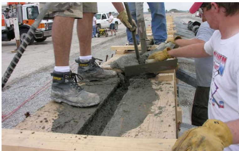
Figure 58. TL-5 Median Barrier Construction
