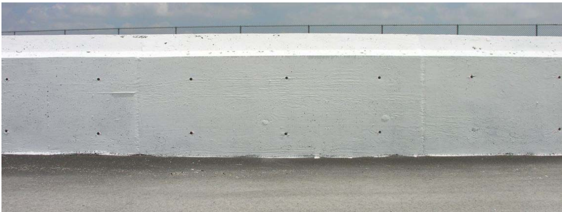
Figure 60. TL-5 Concrete Median Barrier
