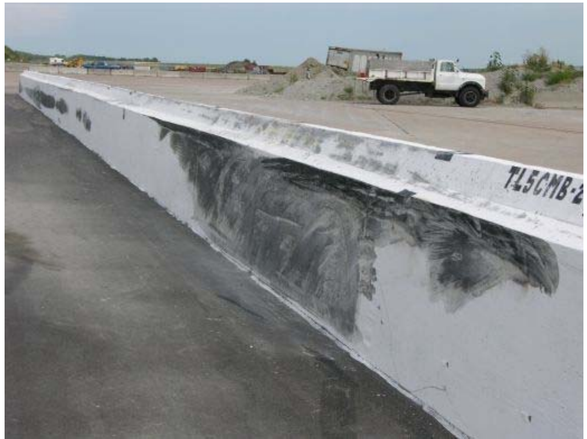
Figure 73. Barrier Damage, Test TL5CMB-2
