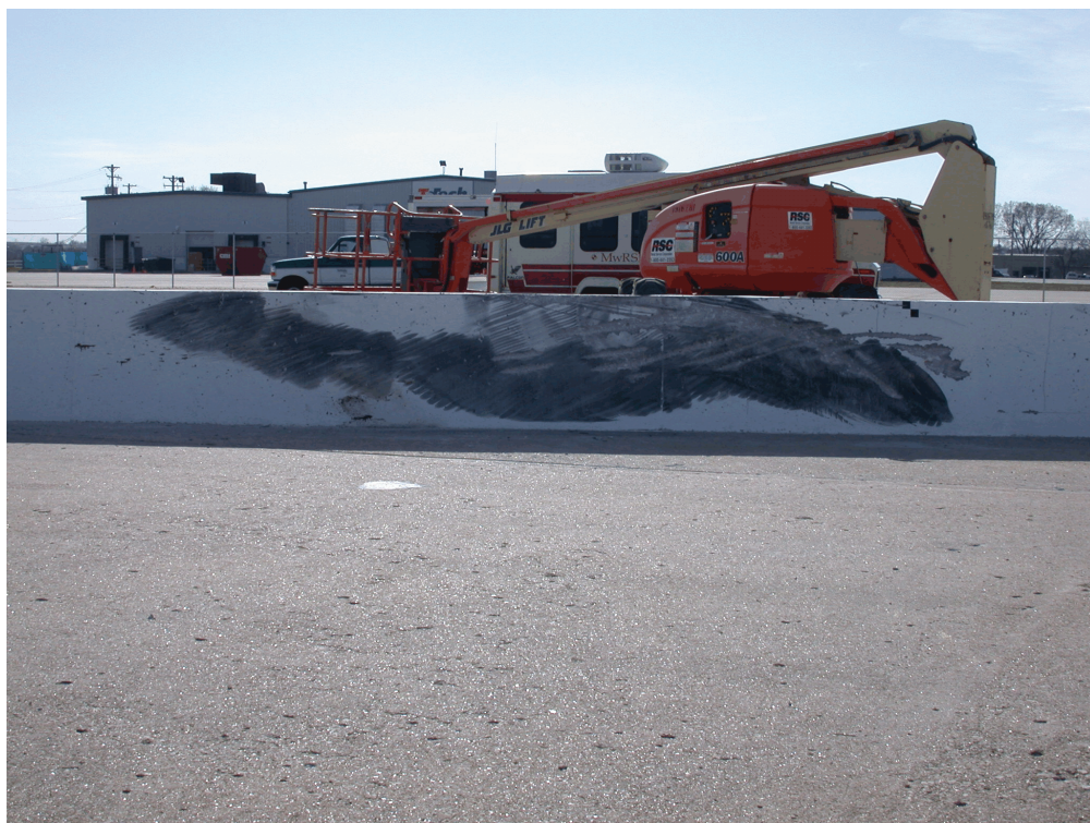
Figure 35. System Damage, Test No. ZOI-1
