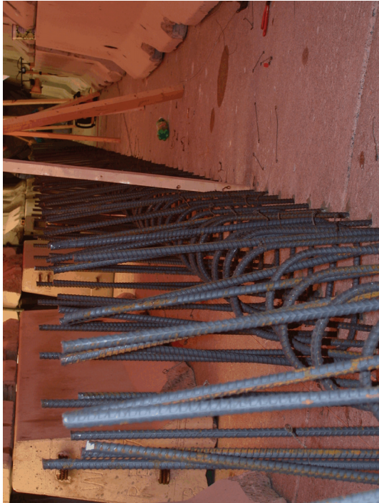
Figure 7. Single-Slope Concrete Barrier Construction
