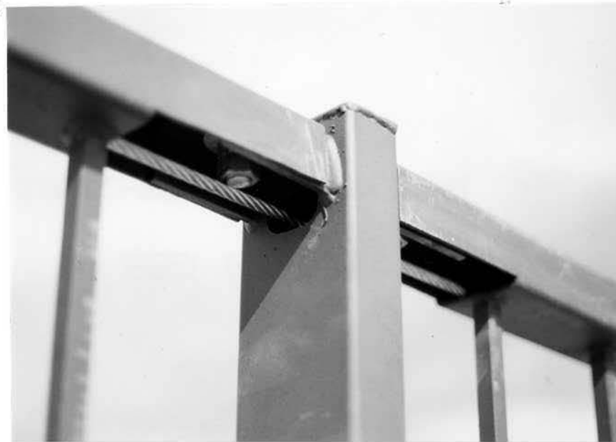
Figure 9. Combination Traffic/Bicycle Bridge Rail
