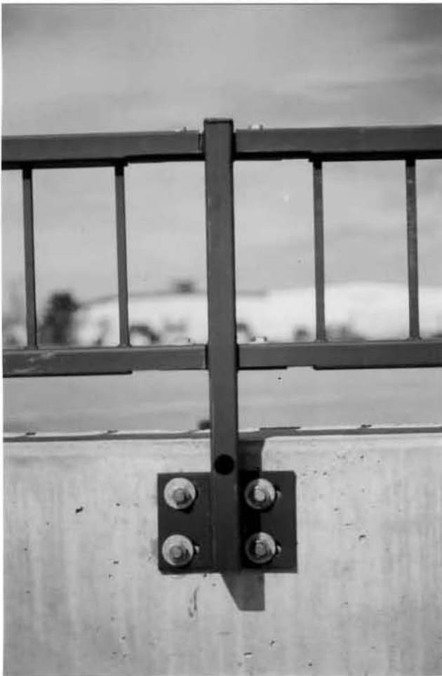
Figure 8. Combination Traffic/Bicycle Bridge Rail
