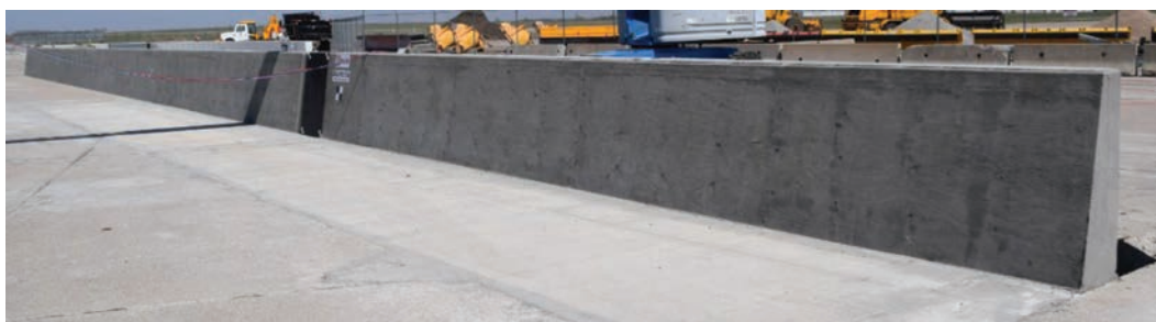
Figure 26. Test installation for Test MAN-1 [Rosenbaugh 2016].
