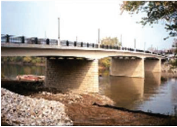
(a) Pier wall
