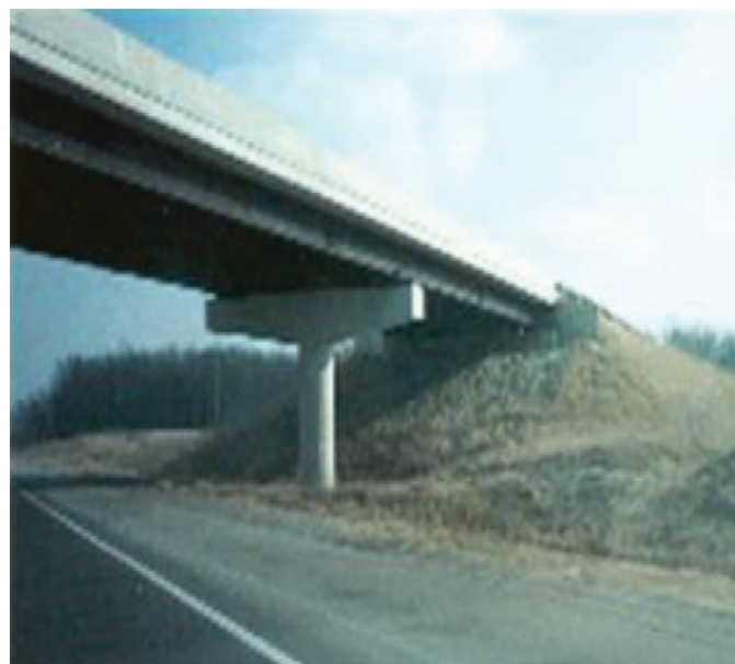
Figure 2. Single-column bridge pier system [ODOT 2014].
