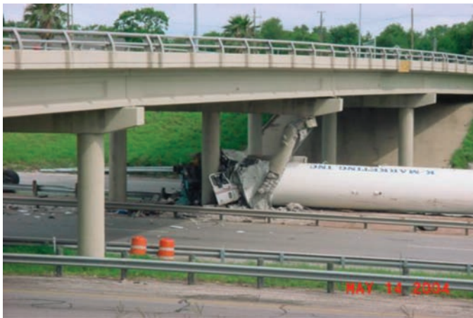
Column-foundation failure
