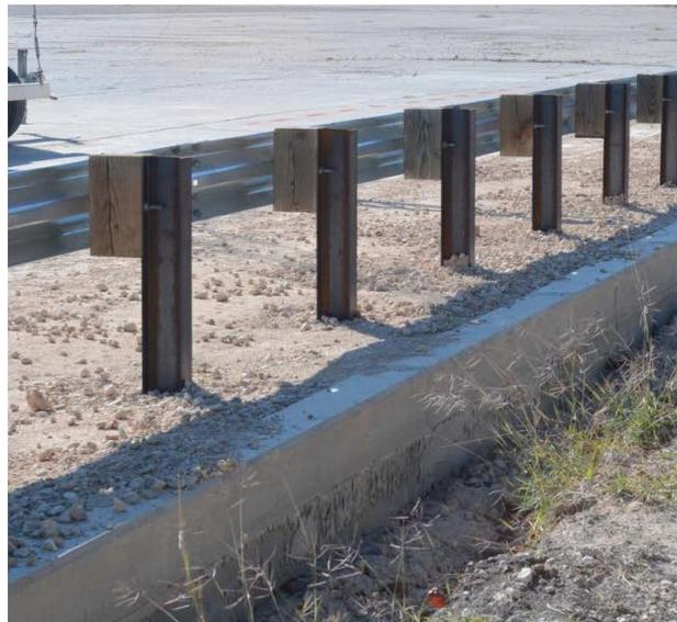
**FIGURE 8 Details and photos of (a) side-mounted and (b) top-mounted guardrail systems attached to culverts.**
