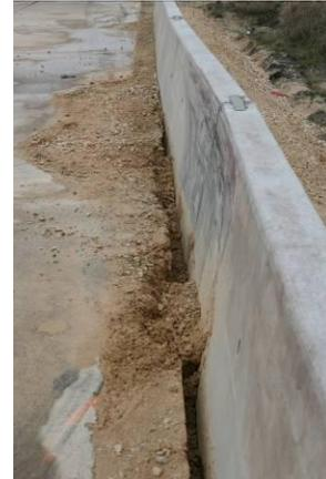
(a) Test article damage
