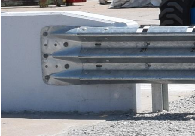
(b) Buttress Connection
