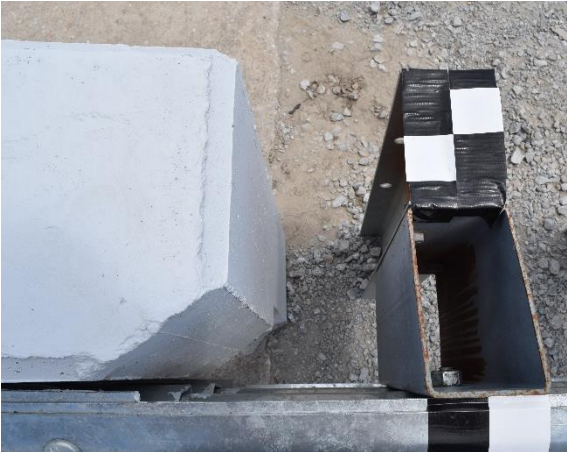
(c) Buttress Overhead
