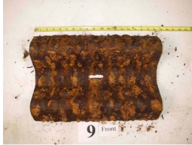
Figure 12 - WSGR Assembled Joint after Exposure
