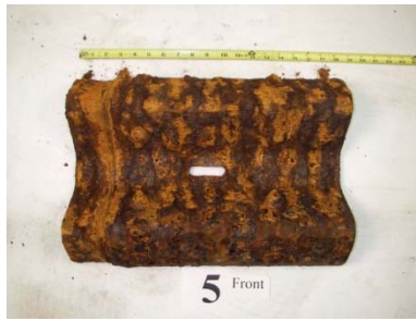
Figure 17 - WSGR with GSGR Insert Assembled Joint after Exposure
