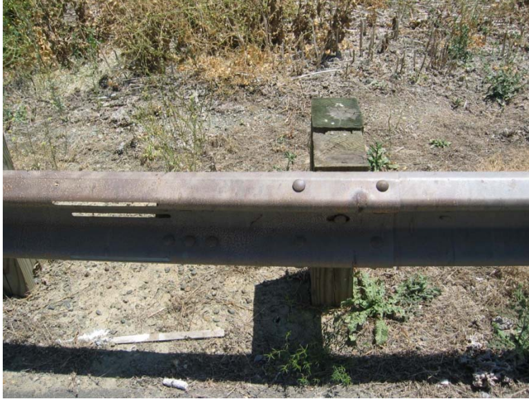
Figure 33 - Staining Product of Galvanized Steel Guardrail
