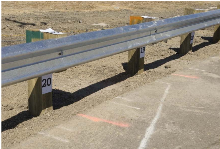
Figure 1 - Galvanized Steel Guardrail
