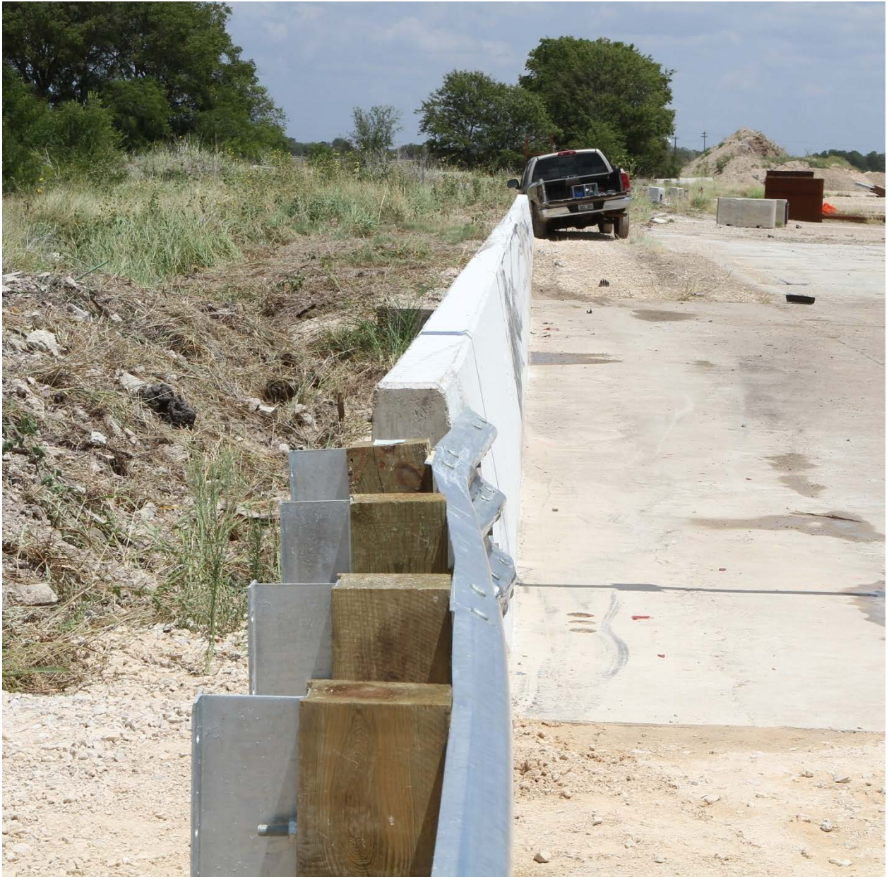
Figure 6.3. Position of Vehicle/Installation after Test No. 420021-4.
