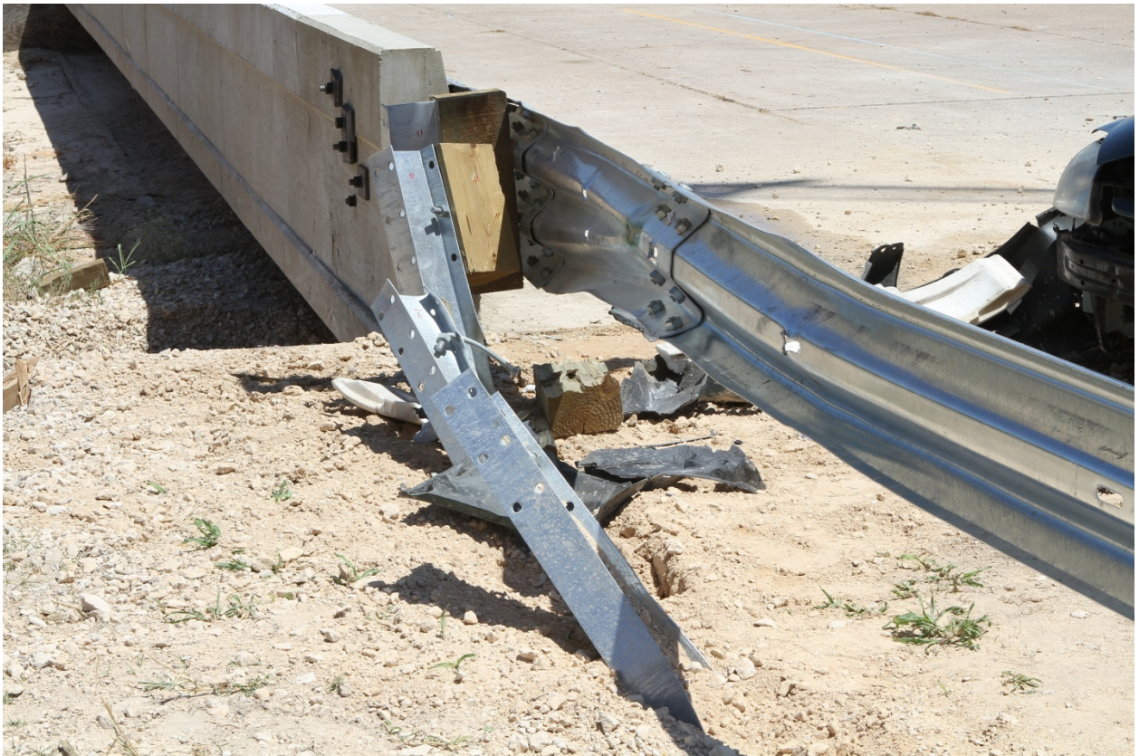
Figure 7.4. Installation after Test No. 420021-6.
