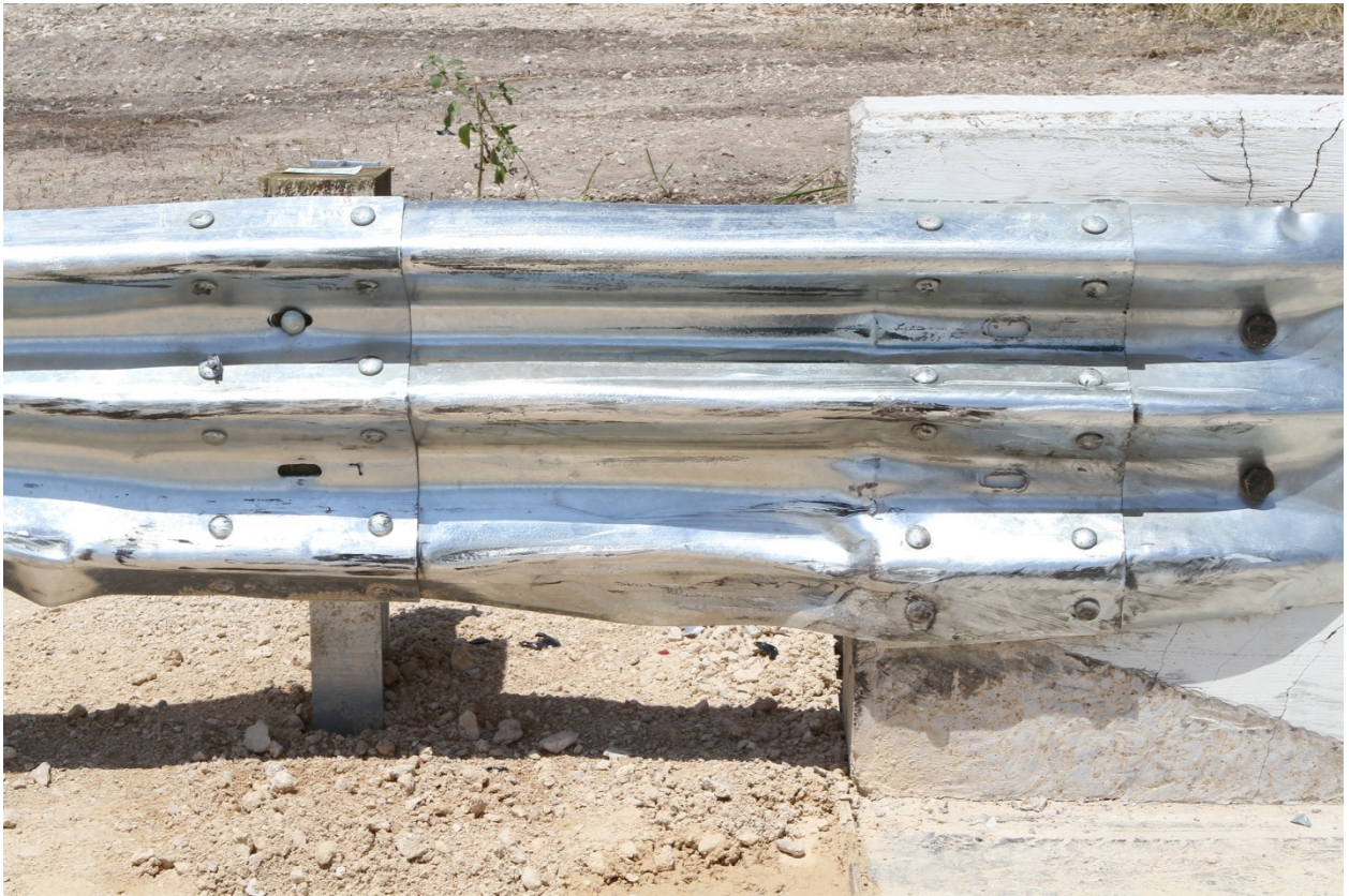
Figure 6.4. Installation after Test No. 420021-4.
