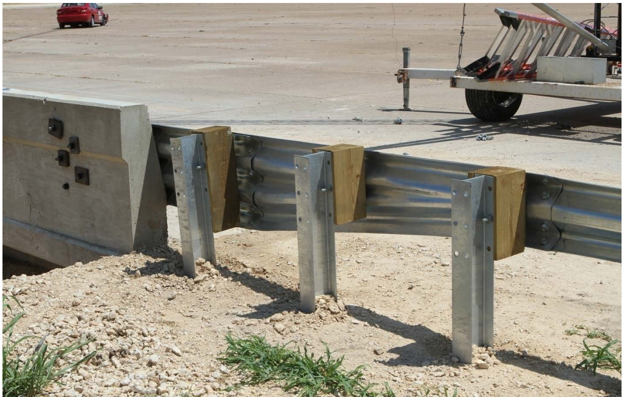
Figure 8.4. Installation after Test No. 420021-7.
