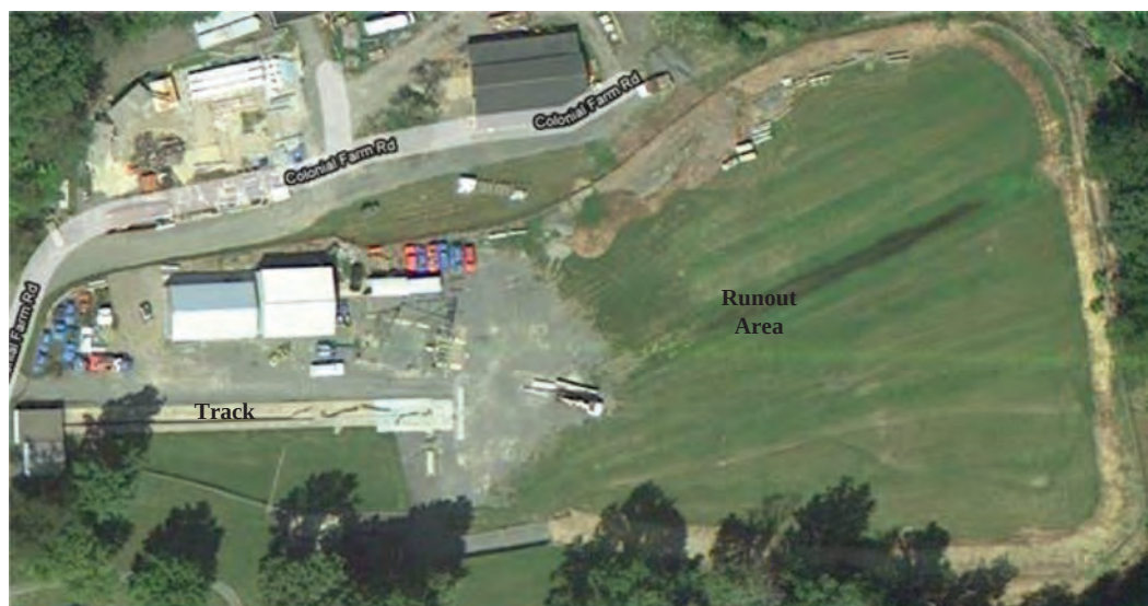
Figure 6.1. Aerial view of the FHWA FOIL facility.
