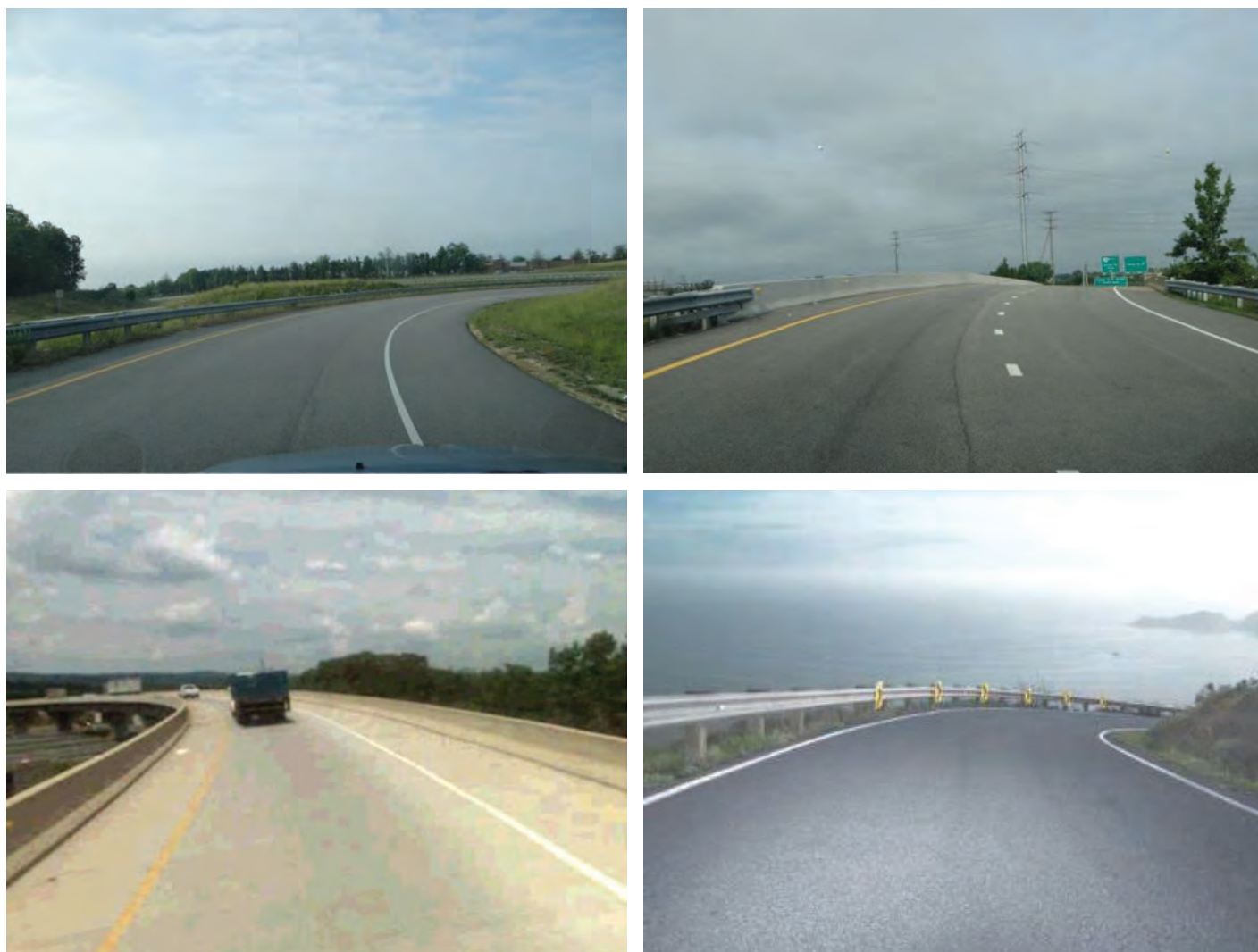
Figure 1.1. Example CSRS with typical longitudinal barriers.
