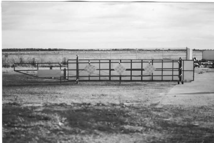
Figure 3. Road Closure Gate
