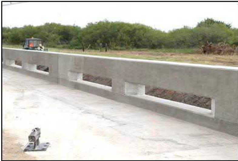
Figure 3.37 TxDOT T224 MASH TL-5 Bridge Rail System (10) .
