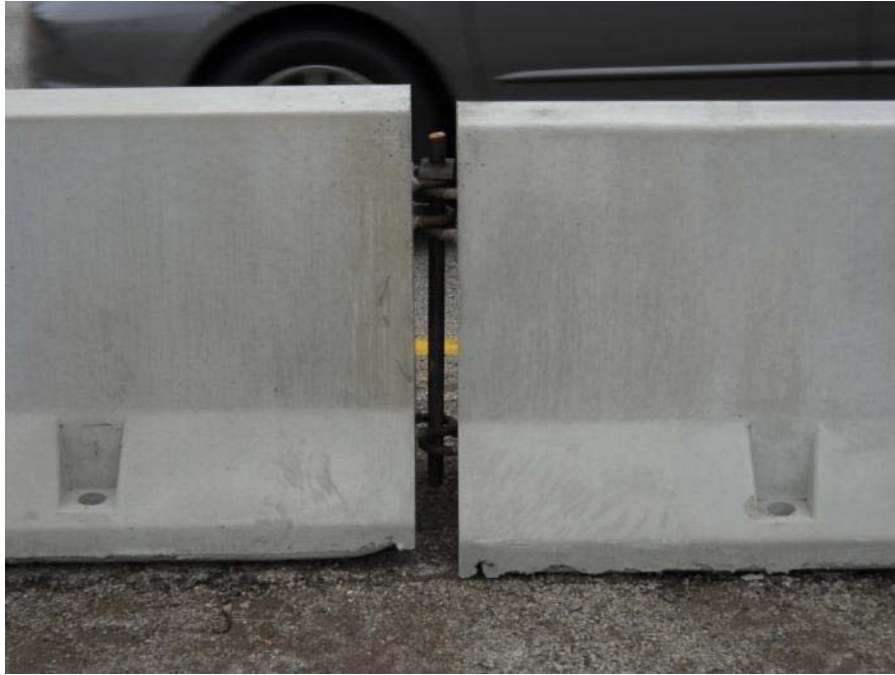
Figure 22 Improper Connection of 12.5' Temporary Barrier
