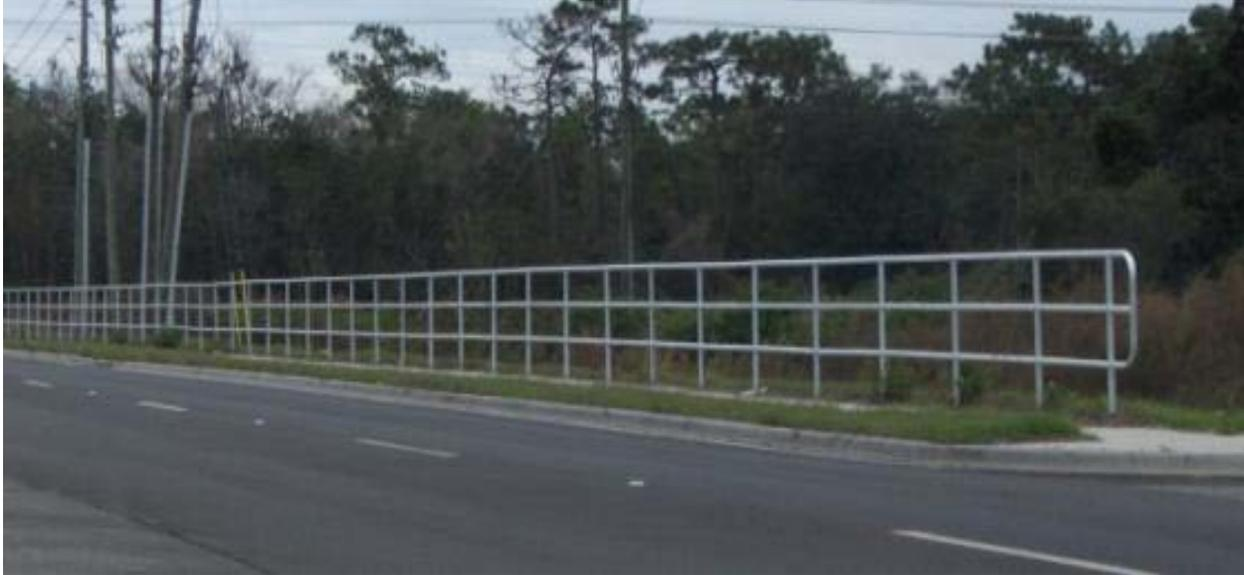
**Figure 2. Pedestrian Rail with Limited Escape Routes from Errant Vehicles**
