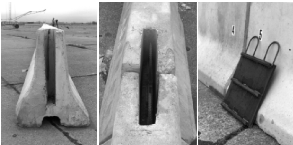
Figure 8: Texas grid-slot connection (Bligh et al., 2002)
