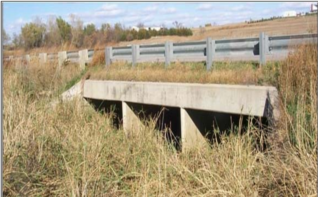
Figure 8. Guardrail installed to shield culvert opening
