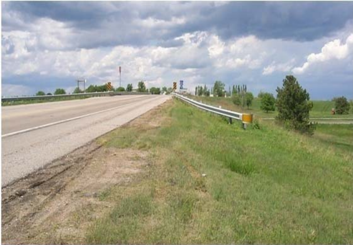
Figure 19. Flared guardrail installation
