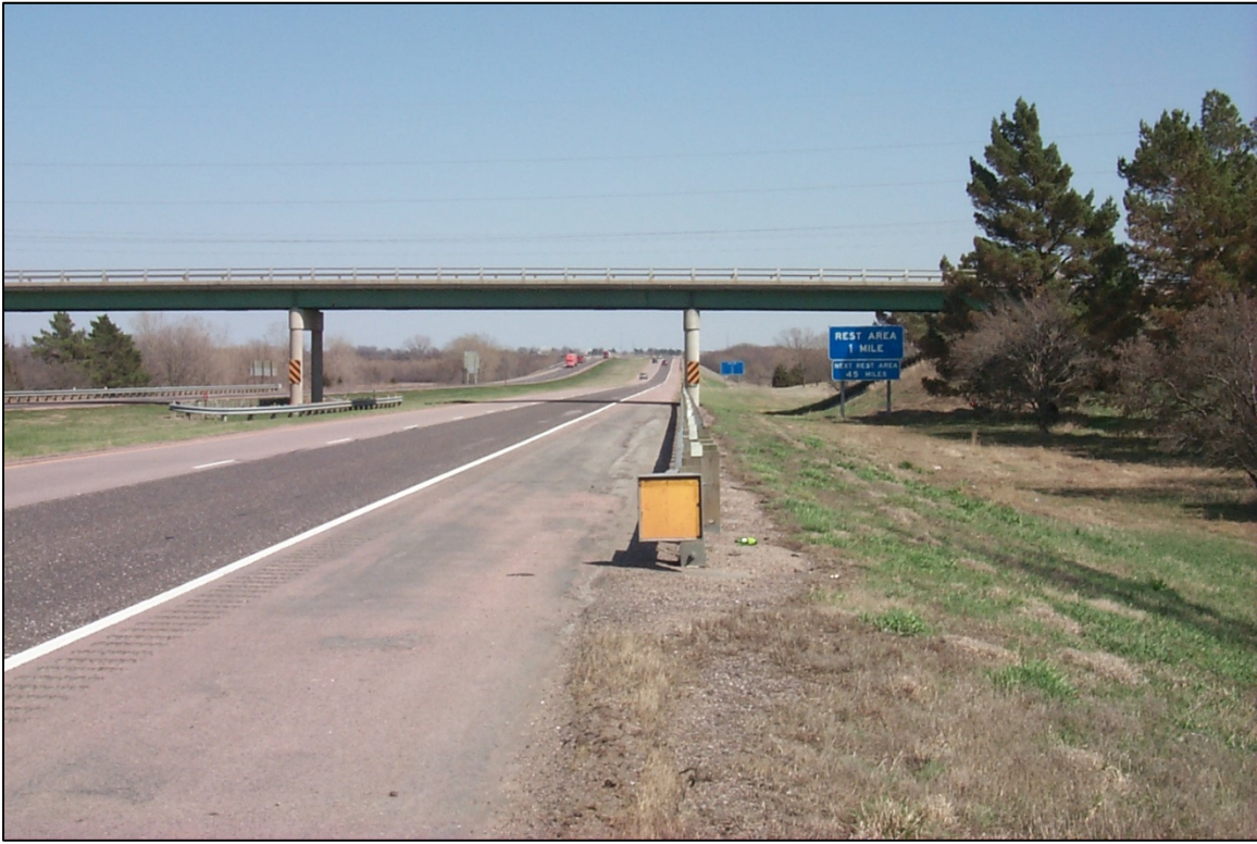
Figure 20. Tangent guardrail installation
