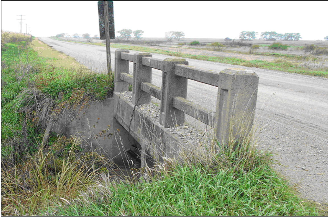
Figure 2. Culvert opening on a local road
