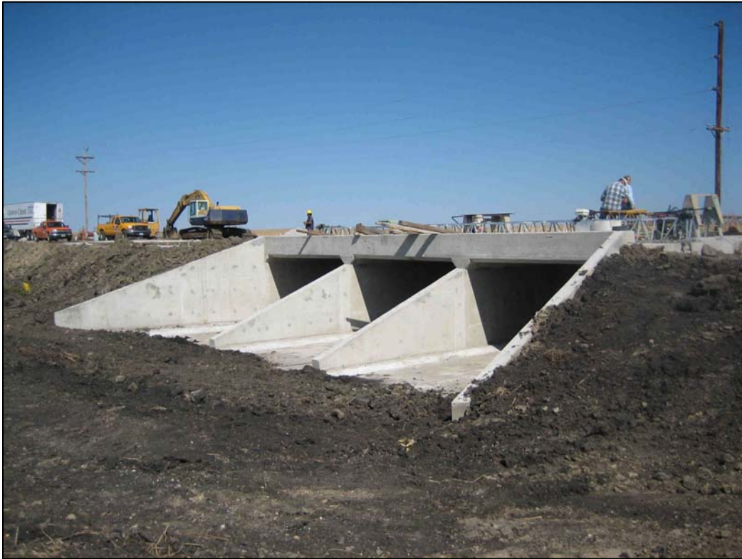
Figure 7. Culvert extension under implementation
