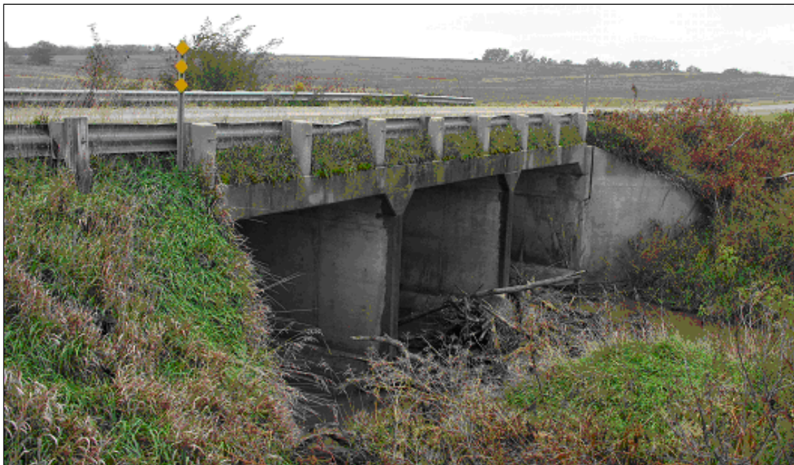
Figure 17. Culvert opening shielded by a guardrail installation
