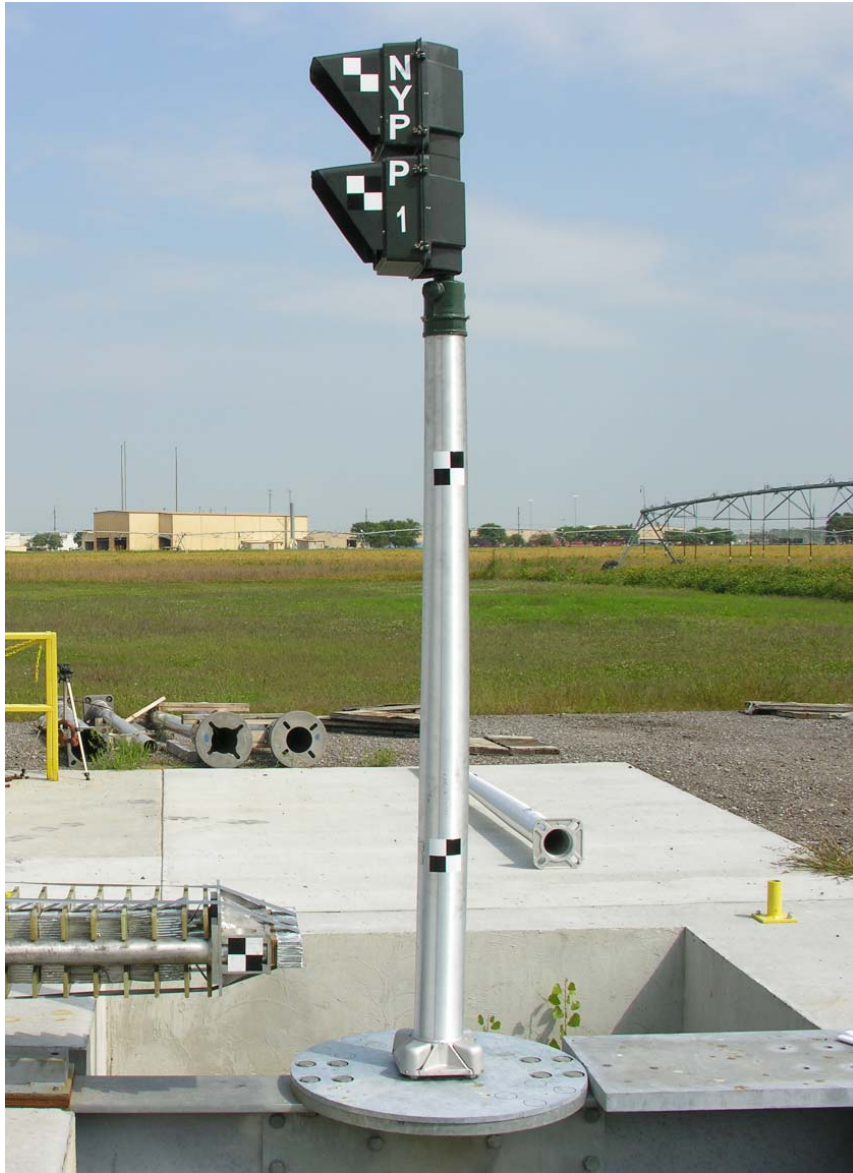
Figure 27. Assembled Pedestrian Signal Test Installation
