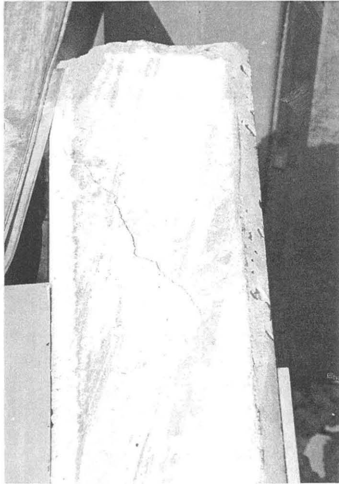
Figure 31. Cracking in Concrete End Section, Test ITNJ-1 (Design No. 1)
