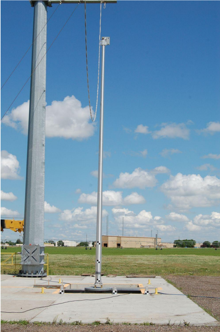
Figure 39. Assembled Test Installation, Test No. BBC-5
