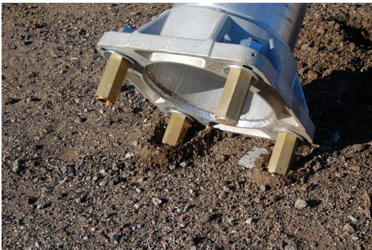
Figure 70. System Damage, Test No. BBC-7
