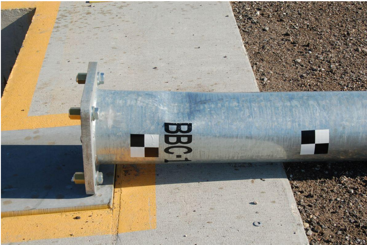
Figure 29. System Damage, Test No. BBC-1
