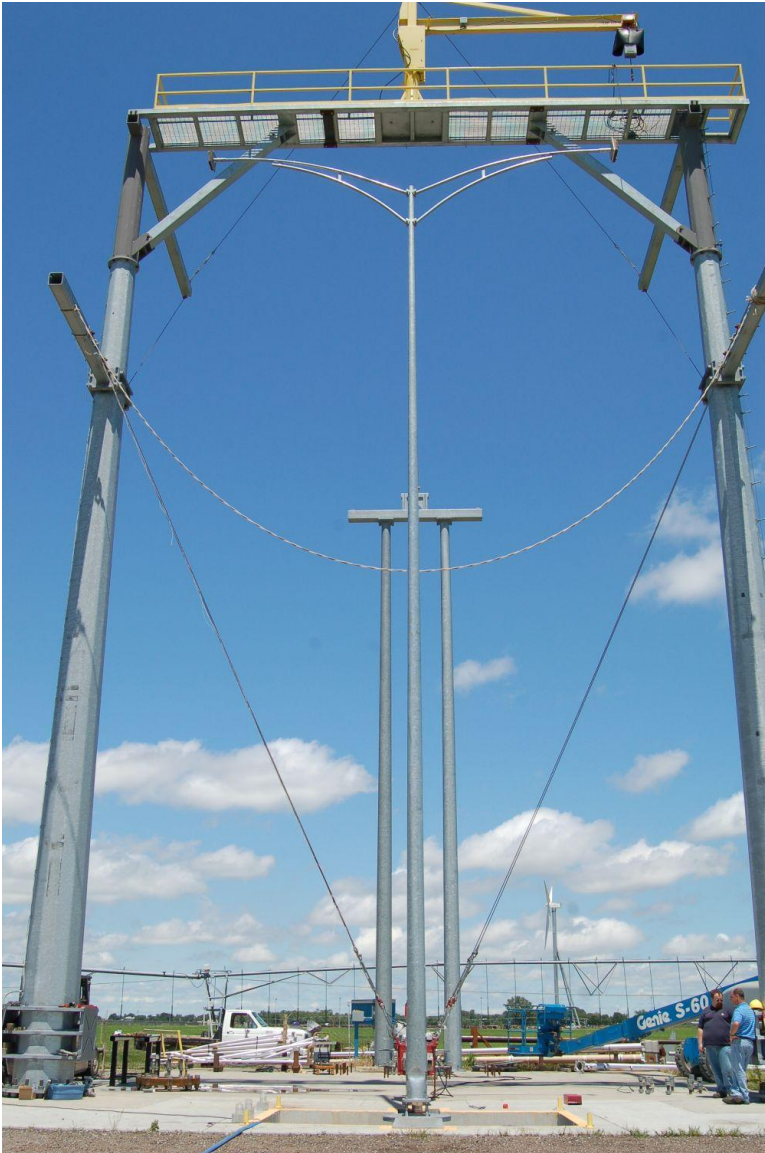
Figure 38. Assembled Test Installation, Test No. BBC-4
