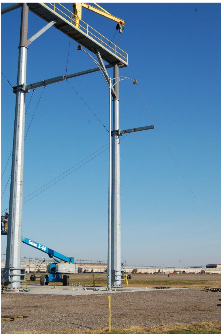
Figure 23. Assembled Test Installation, Test No. BBC-1
