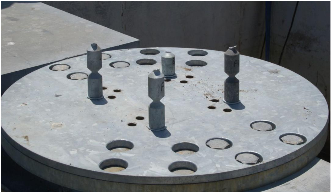
Figure 48. System Damage, Test No. BBC-4
