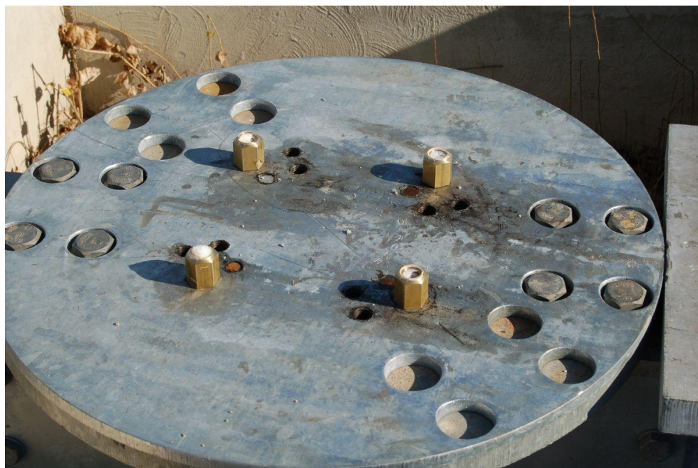
Figure 28. System Damage, Test No. BBC-1
