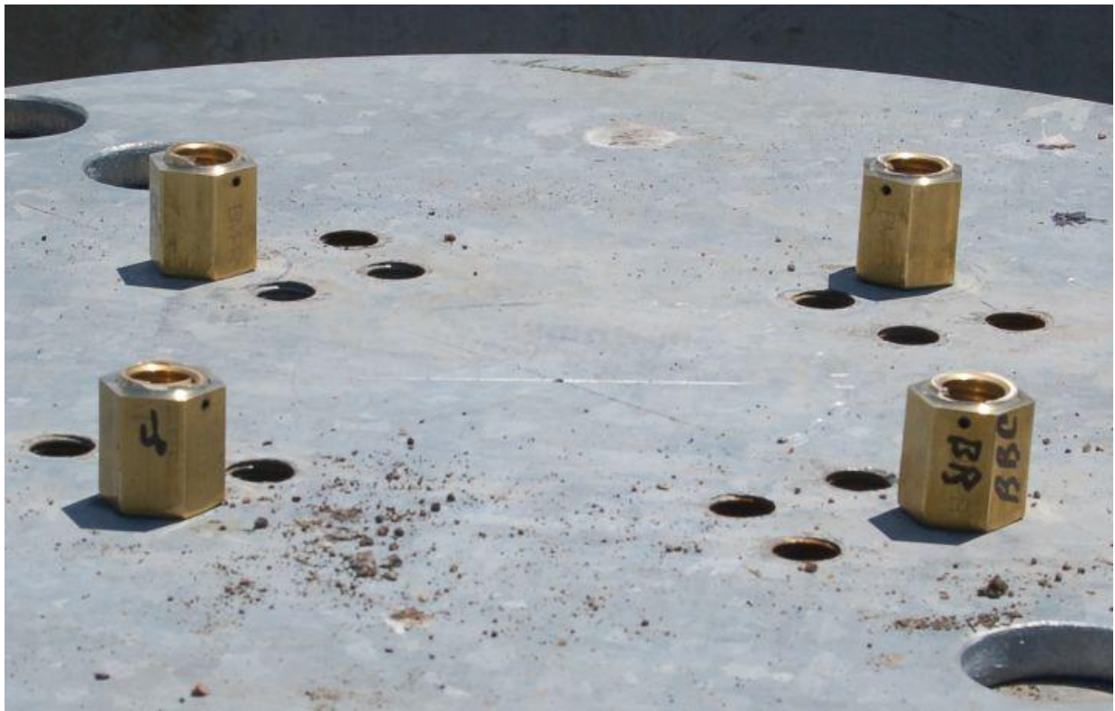
Figure 44. System Damage, Test No. BBC-3
