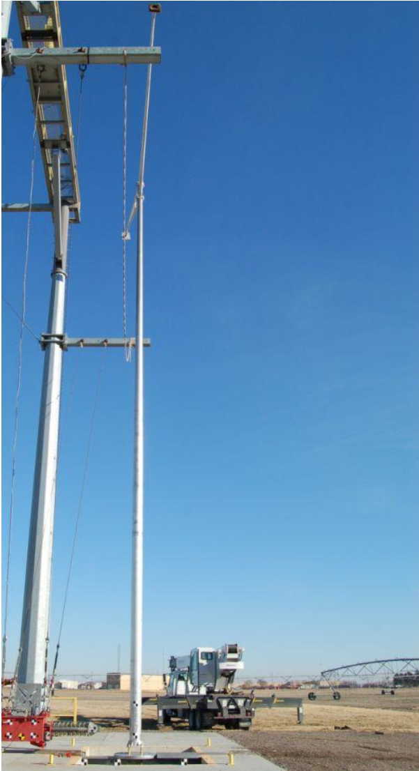
Figure 60. Assembled Test Installation, Test No. BBC-7
