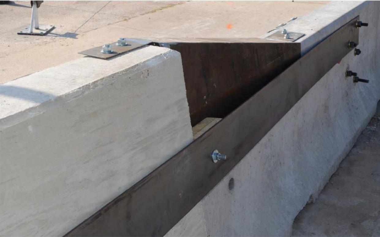
Figure 4. Transition Design for Anchored Temporary Barrier to Rigid Concrete Barrier [12]
