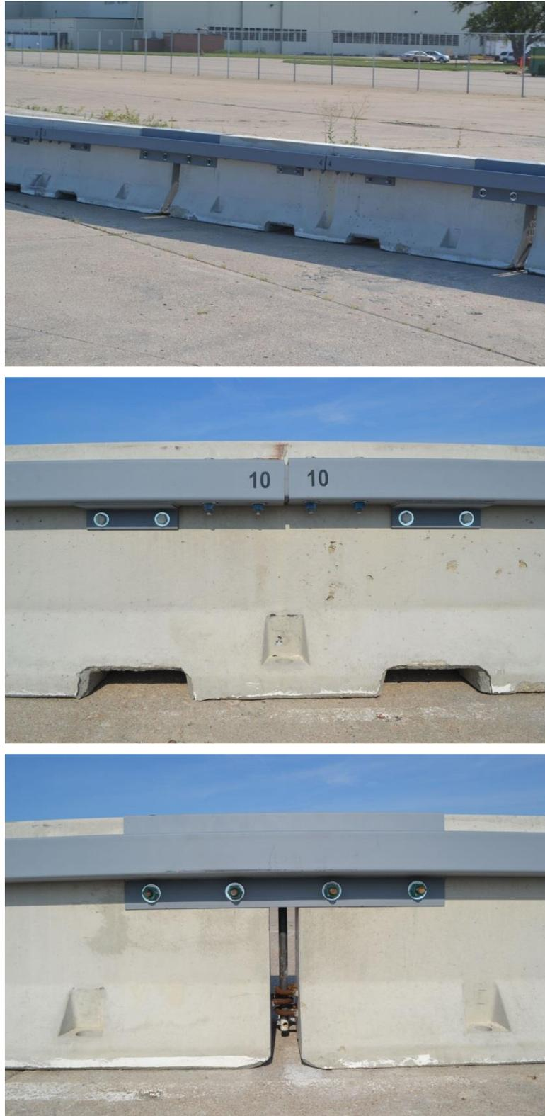
Figure 1. WisDOT Modified Reduced-Deflection Portable Concrete Barrier [5]
