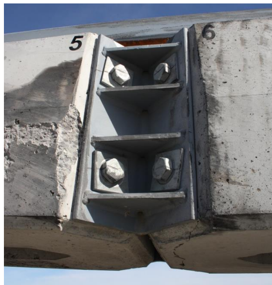
Figure 112. System Damage, Post Contact and Joint between Barrier Nos. 5 and 6, Test No. SFH-3
