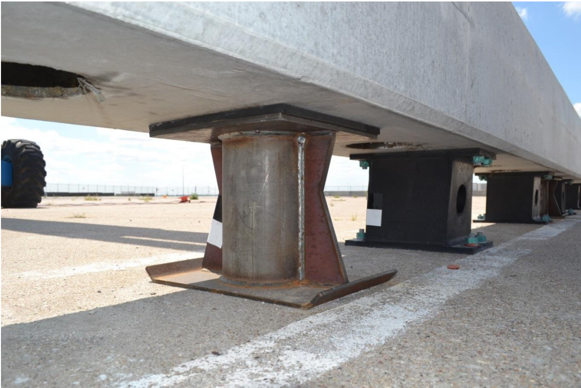
Figure 28. Test Installation Photographs, Skids and Upper Tube Assembly Splices, Test Nos. SFH-1 through SFH-2
