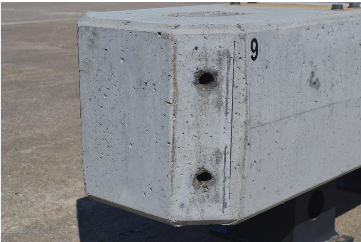
Upstream Barrier No. 9
