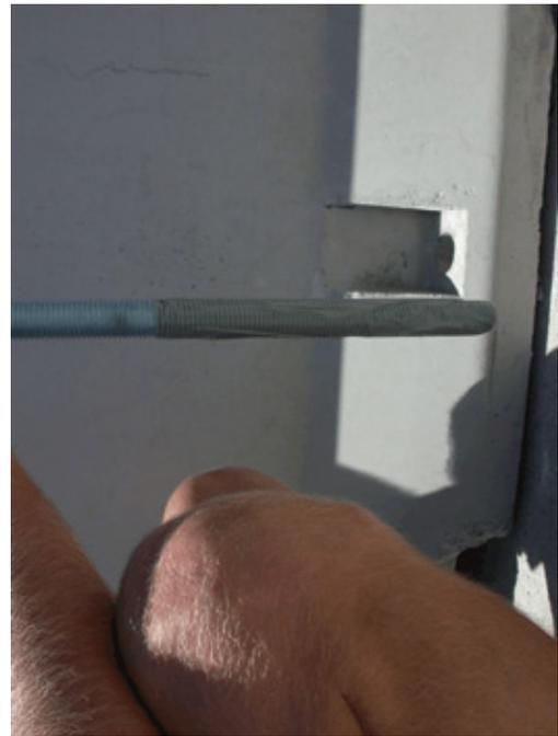
Figure 11. Barrier Tie-Down Installation
