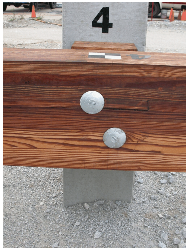
Figure 14. Mn/DOT's Timber Rub Rail Design for Noise Barriers
