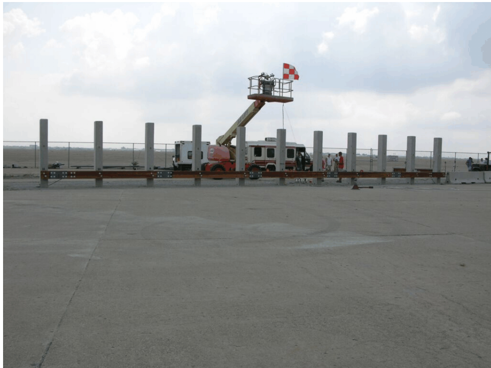
Figure 12. Mn/DOT's Timber Rub Rail Design for Noise Barriers
