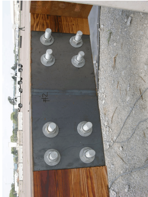
Figure 15. Mn/DOT's Timber Rub Rail for Noise Barriers
