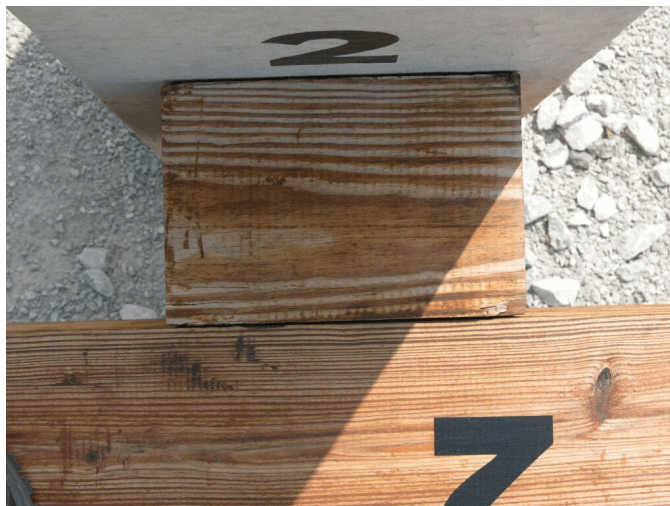
Figure 16. Mn/DOT's Timber Rub Rail Design for Noise Barriers
