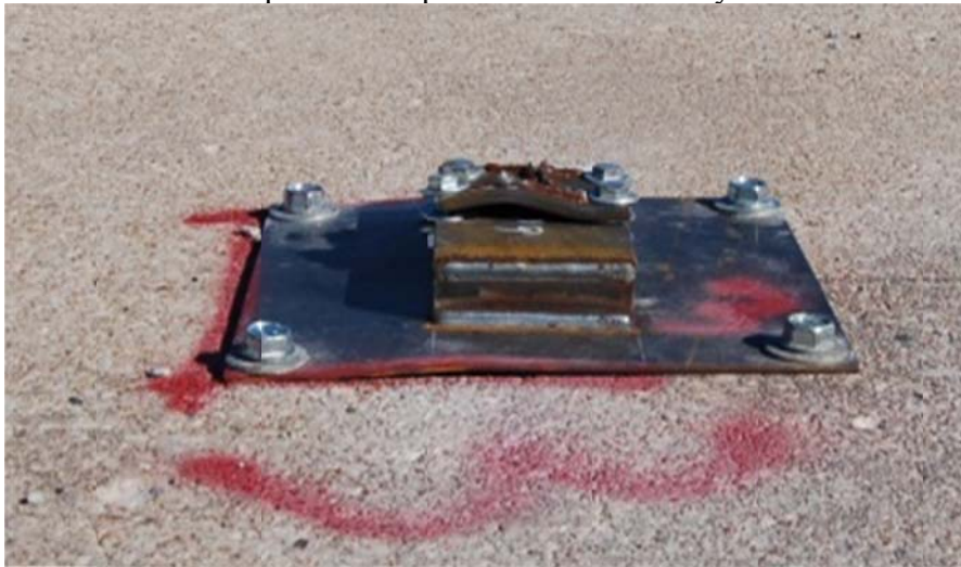
Upstream Slip Base Post Assembly
