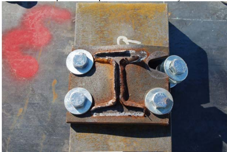
Upstream Slip Base Post Assembly
