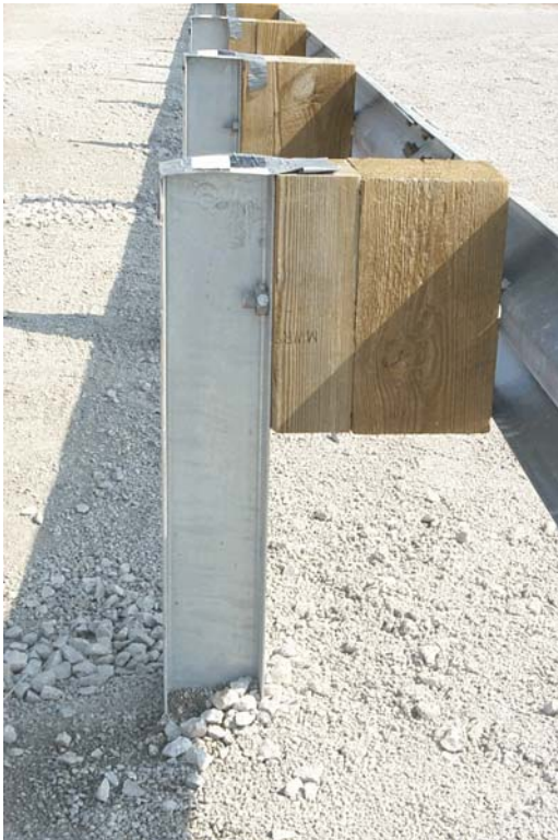
Figure 54. Midwest Guardrail System Nominal Height
