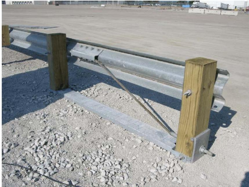
Figure 21. Approach Guardrail Transition to Concrete Barrier System
