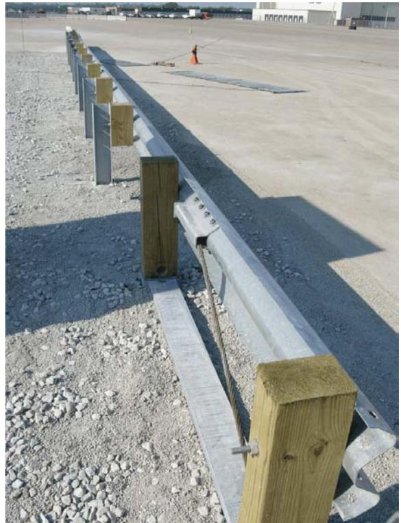
Figure 20. Approach Guardrail Transition to Concrete Barrier System
