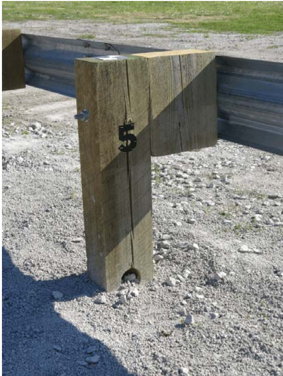
Figure 22. Midwest Guardrail System End Terminal
