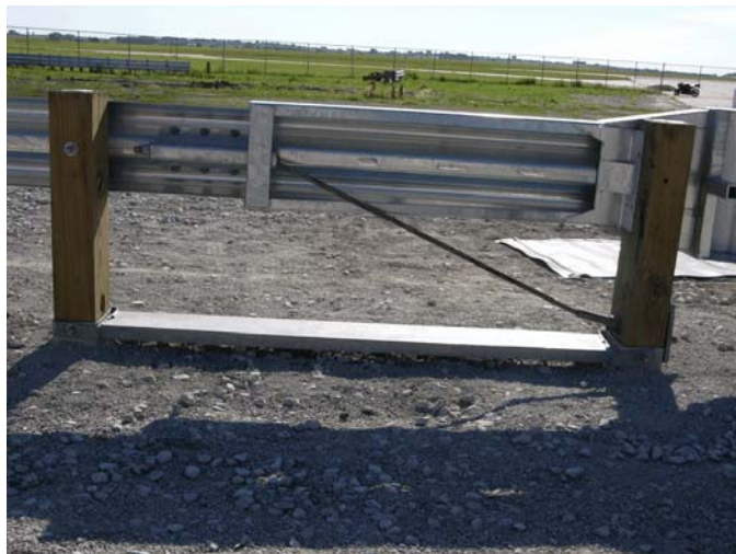
Figure 20. Midwest Guardrail System End Terminal
