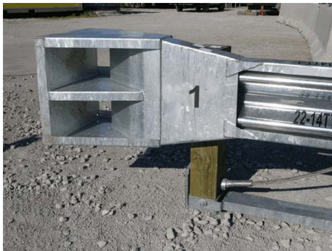
Figure 21. Midwest Guardrail System End Terminal
