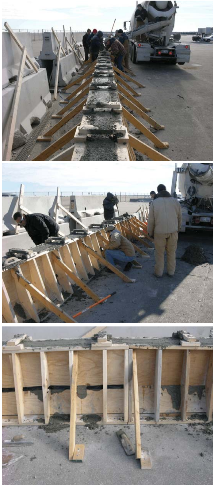
Figure 10. Permanent New Jersey Safety Shape Barrier System Construction
