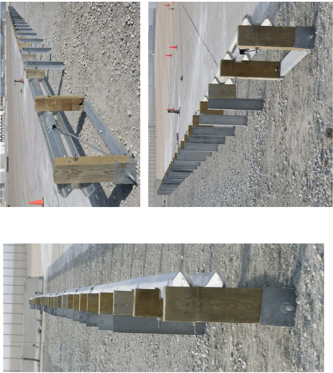
Figure 12. Standard Height, Strong Post, Wood Blockout W-Beam Guardrail System
