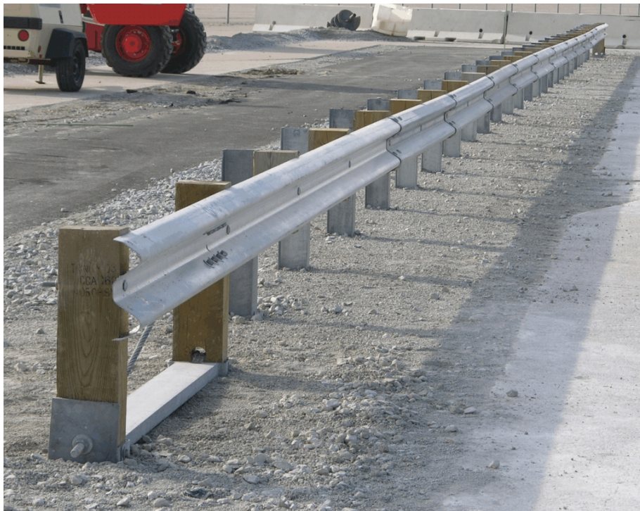
Figure 11. Standard Height, Strong Post, Wood Blockout W-Beam Guardrail System
