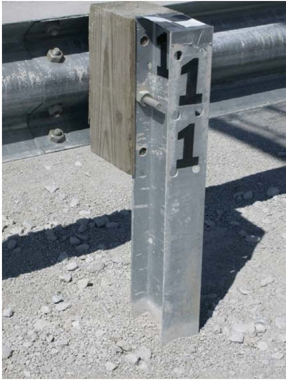
Figure 13. Standard Height, Strong Post, Wood Blockout W-Beam Guardrail System
