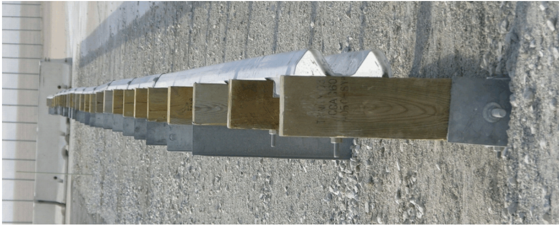
Figure 12. Standard Height, Strong Post, Wood Blockout W-Beam Guardrail System
