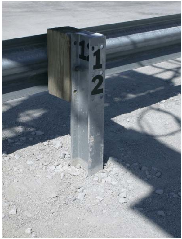
Figure 13. Standard Height, Strong Post, Wood Blockout W-Beam Guardrail System
