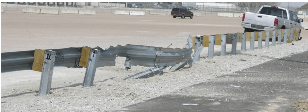
Figure 23. Standard Strong-Post, WoodBlockout, W-beam Guardrail System Damage, Test 2214WB-2
