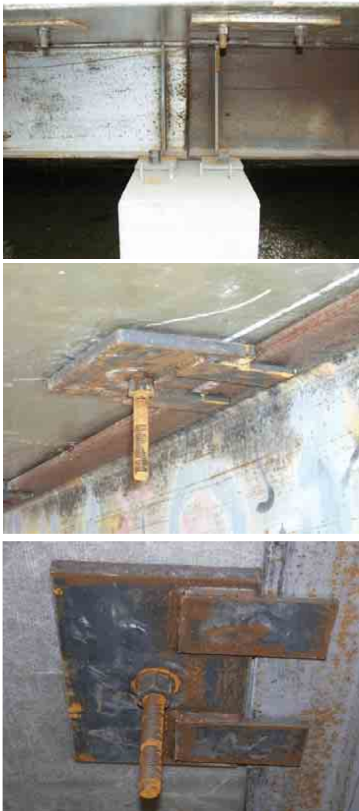
Figure 15. Composite Deck Panel Connection
