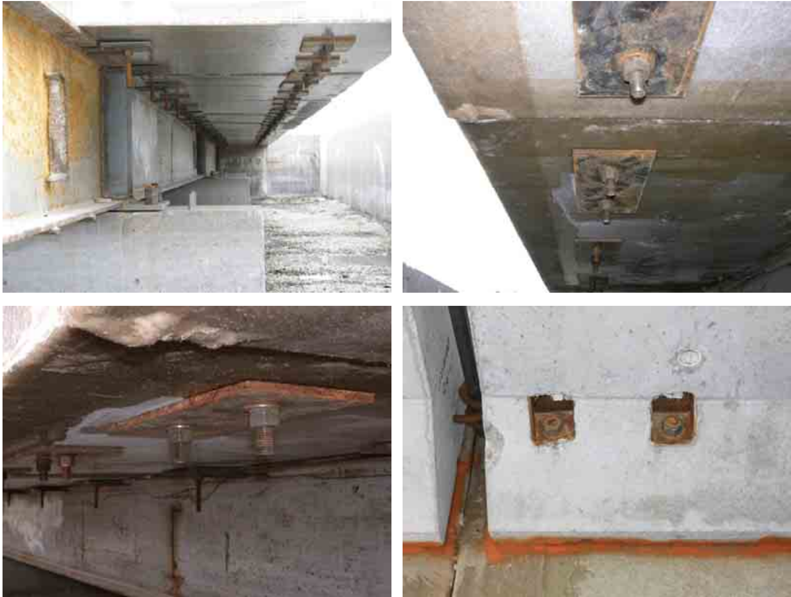
Figure 16. Barrier Anchorage System
