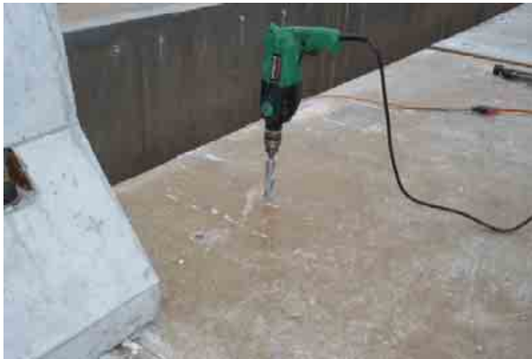
Figure 17. Barrier Attachment to Composite Bridge Deck Installation
