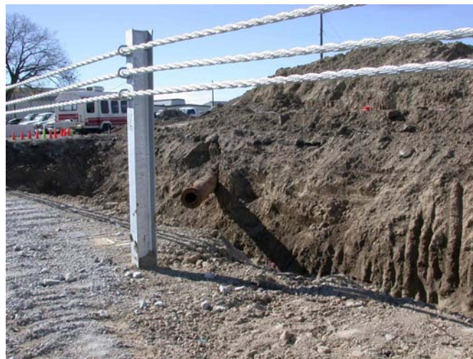
Figure 19. Three-Cable Guardrail System Adjacent to Slope
