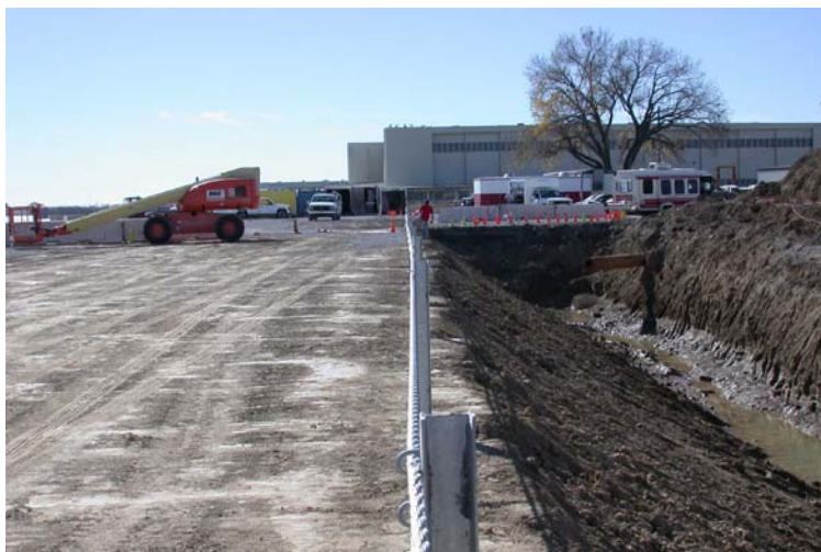
Figure 18. Three-Cable Guardrail System Adjacent to Slope
