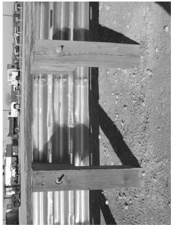
Figure 40. Short-Radius Post Details
