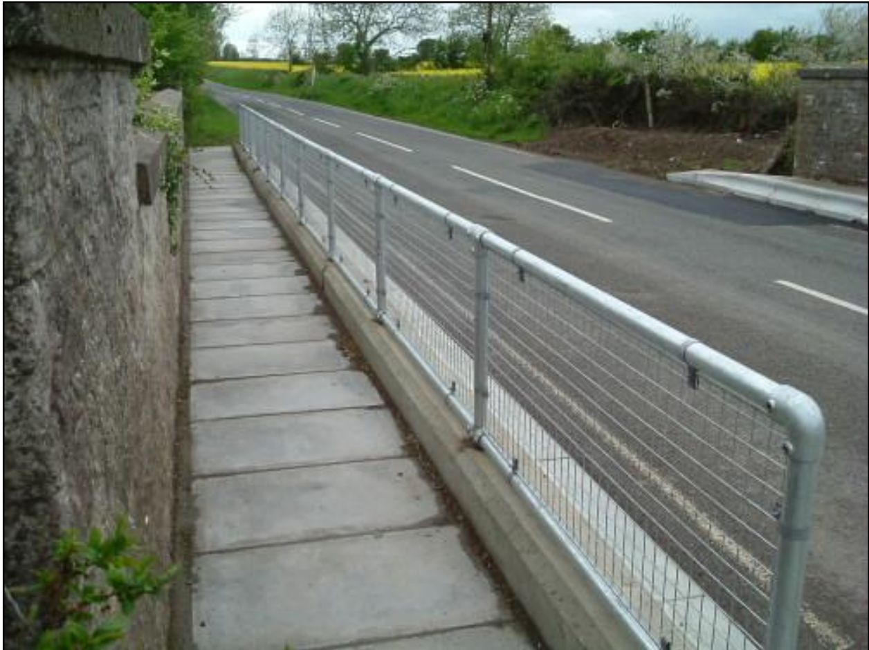
Figure 16: Handrail Separating Sidewalk And Roadway 24
