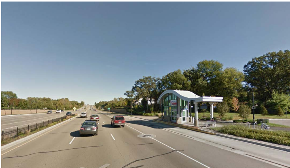
FIGURE 3-20: RED LINE, 140TH STREET STATION, WESTBOUND
