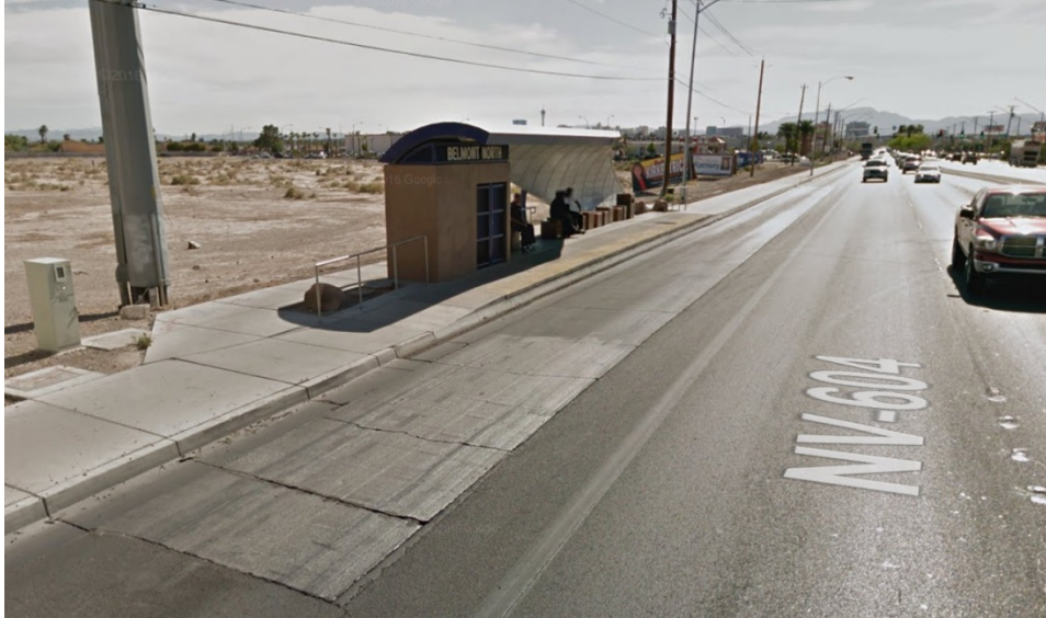
FIGURE 3-2: MAX/ROUTE 113, BELMONT NORTH STATION, LAS VEGAS BOULEVARD NORTH AT BELMONT STREET, NORTHBOUND
