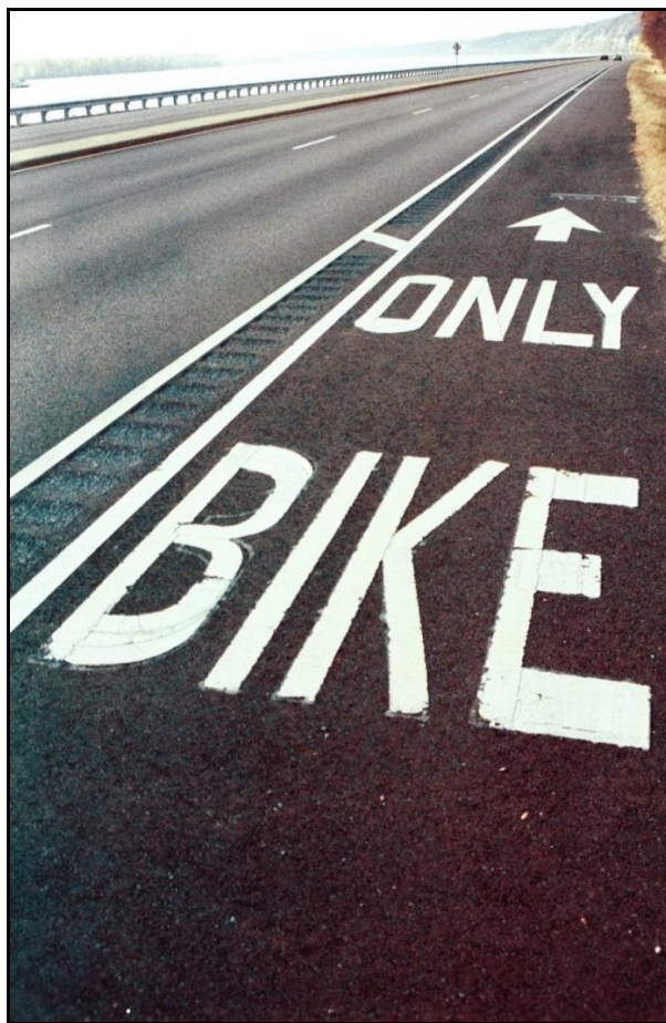
Figure 25: Shoulder Rumble Strips Between Roadway And Bike Lane 32
