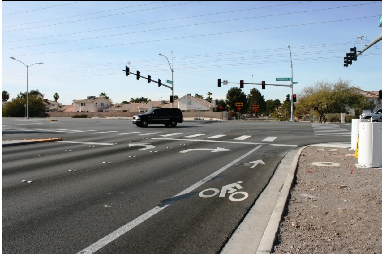
Figure 21: Bicycle Lane Within The Roadway
