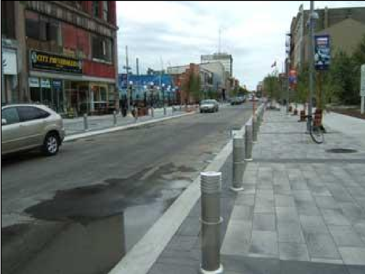
Figure 15: Bollards Separating The Roadway And The Sidewalk 23
