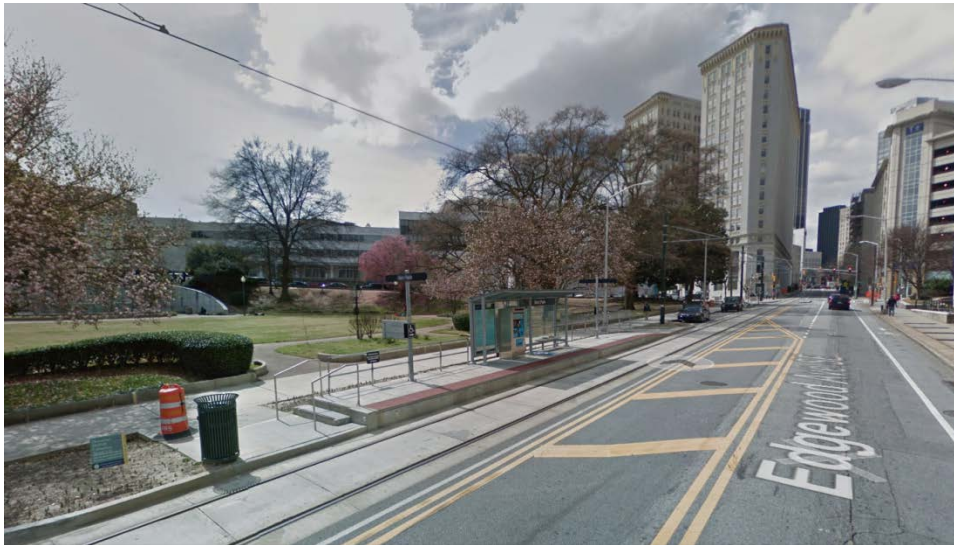
FIGURE 3-32: ATLANTA STREETCAR, HURT PARK STATION, EASTBOUND
