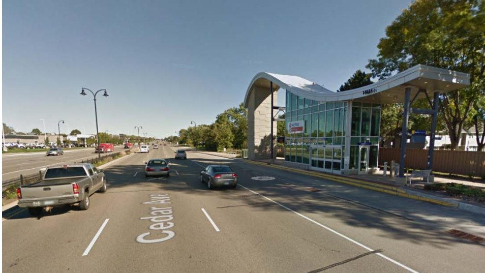
FIGURE 3-21: RED LINE, 147TH STREET STATION, WESTBOUND
