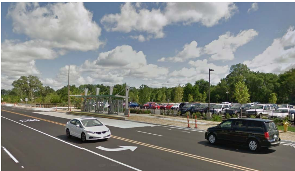
FIGURE 3-14: SILVER LINE, 60TH STREET STATION, NORTHBOUND
