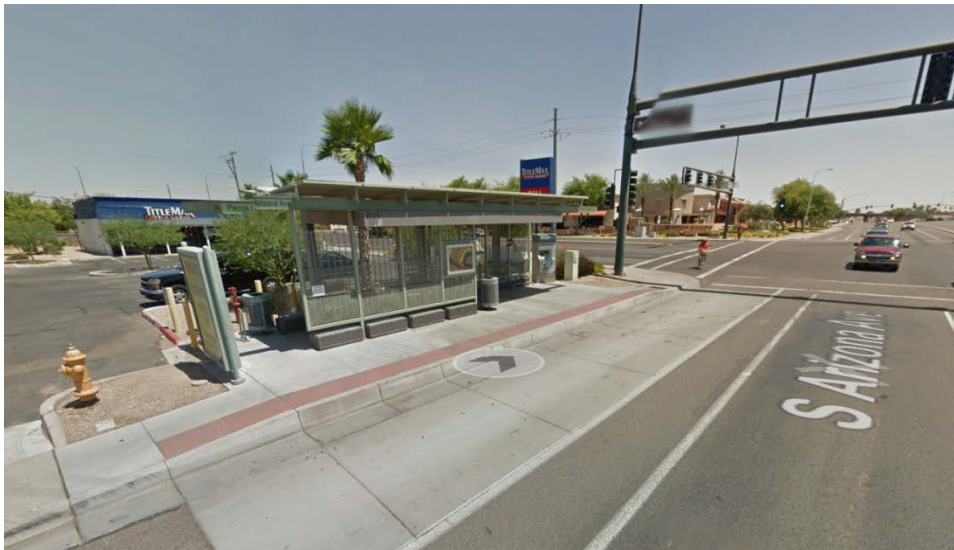
FIGURE 3-11: PECOS ROAD STATION, NORTHBOUND
