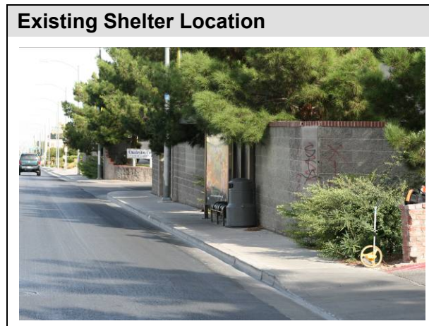
Figure 9. Longitudinal Shelter Relocation
