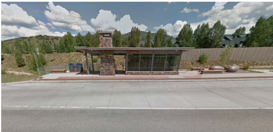
FIGURE 3-28: VELOCIRFTA, BUTTERMILK STATION, NORTHBOUND
