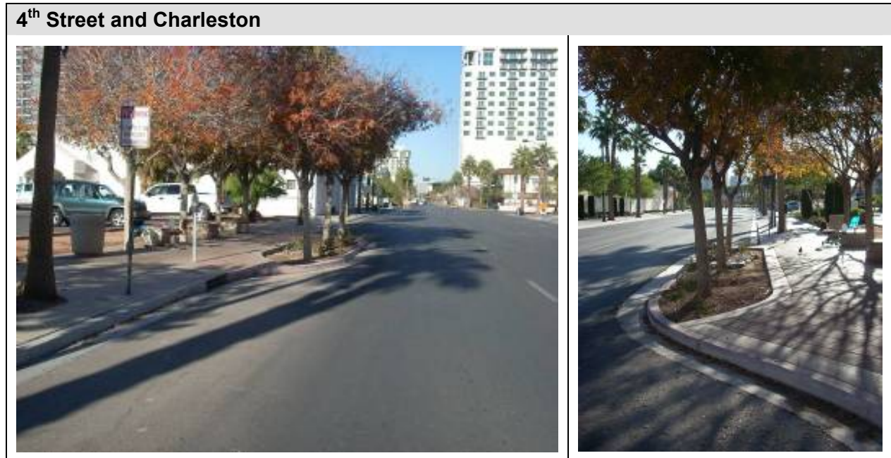
Figure 17. Curb Extension (Bulb-Out)
