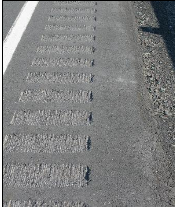
Figure 24: Shoulder Rumble Strips 31
