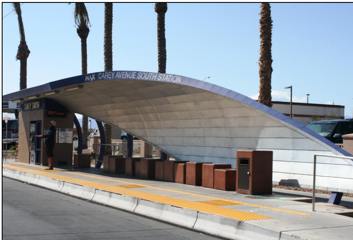
Figure 10: Raised Curb At Las Vegas MAX Stop
