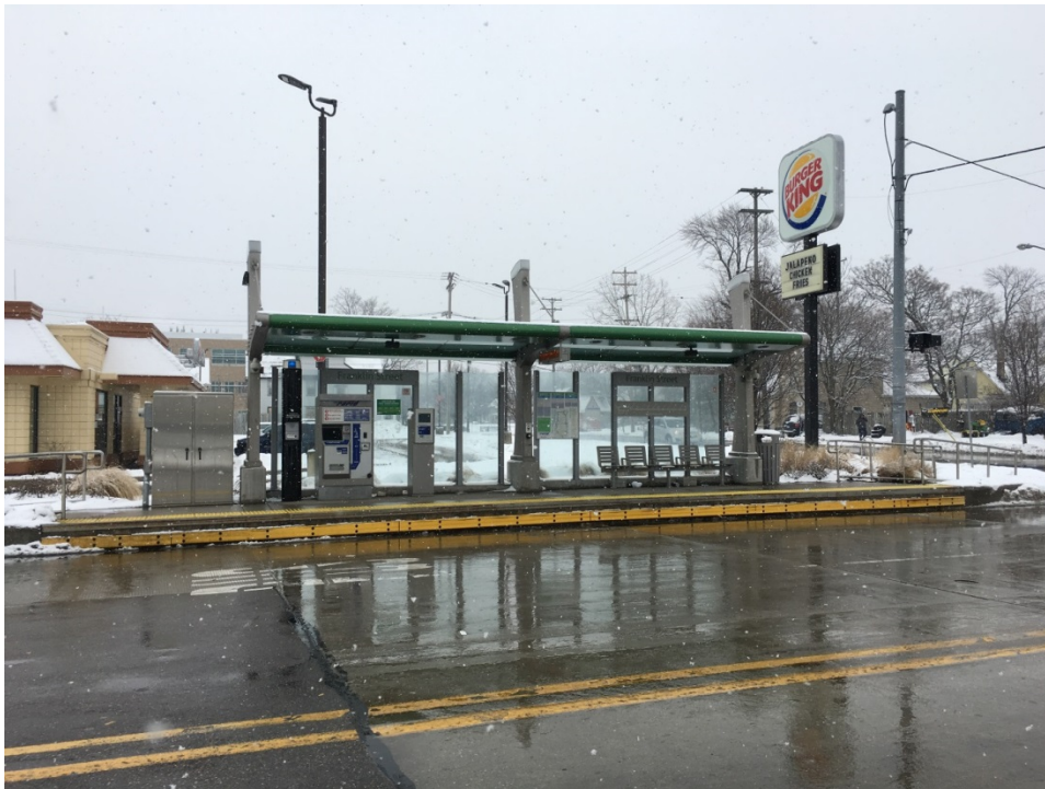
FIGURE 3-16: SILVER LINE, FRANKLIN STREET STATION, NORTHBOUND
