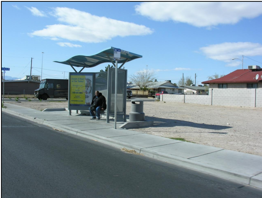
Figure 6: Las Vegas Valley Bus Shelter Located On Bus Pad Behind Sidewalk
