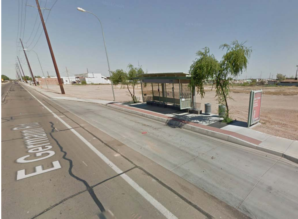
FIGURE 3-12: GERMANN ROAD STATION, EASTBOUND
