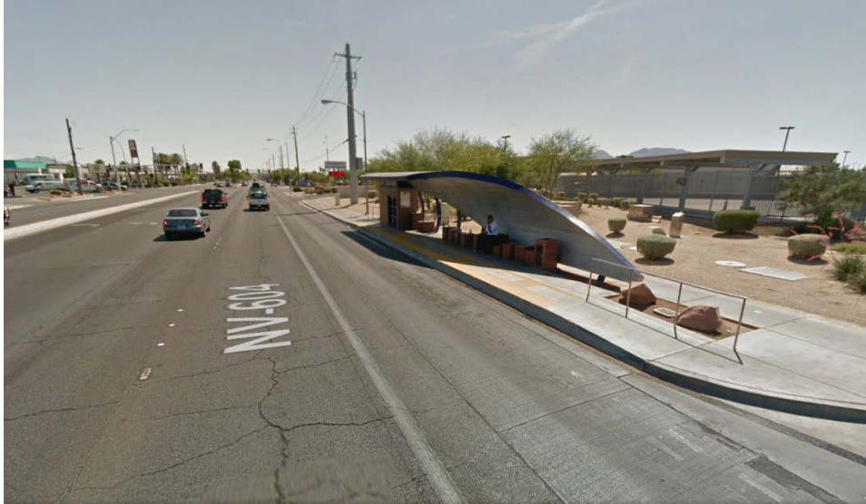
FIGURE 3-4: MAX/ROUTE 113, LAS VEGAS BOULEVARD NORTH AT CIVIC CENTER DRIVE, NORTHBOUND
