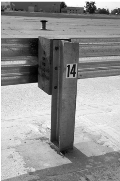
Figure 63. Mow Strip Installation before Test 441622-1.
