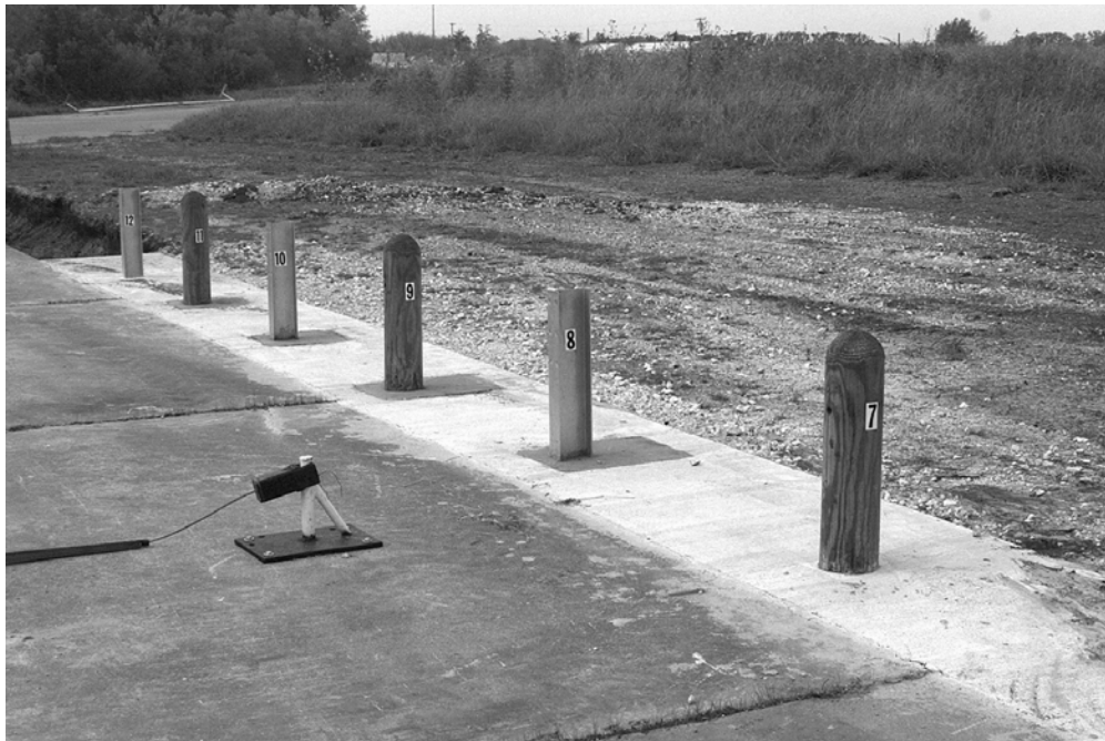
Figure 17. Concrete Mow Strip Test Installation.
