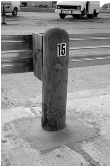
Figure 72. Mow Strip Installation before Test 441622-2.
