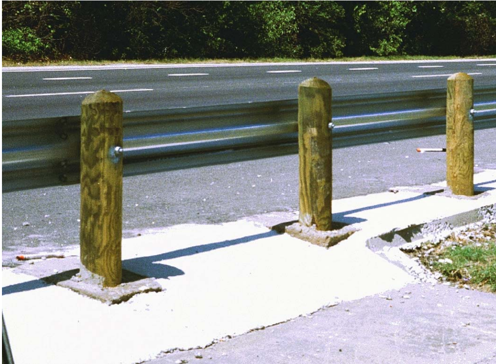
Figure 3. Concrete Mow Strip System with Grout Leave-outs.
