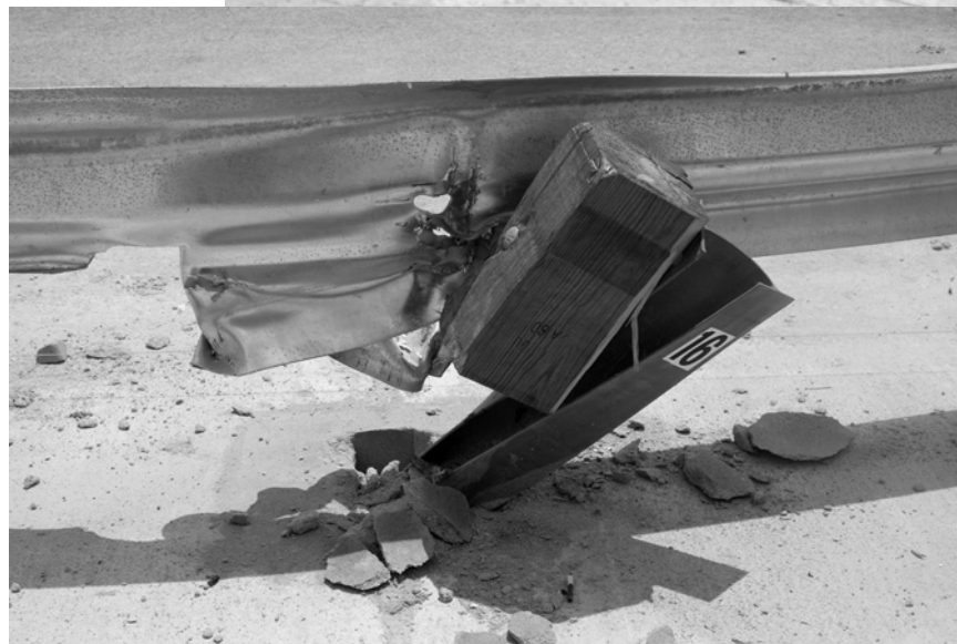
Figure 67. Installation after Test 441622-1.
