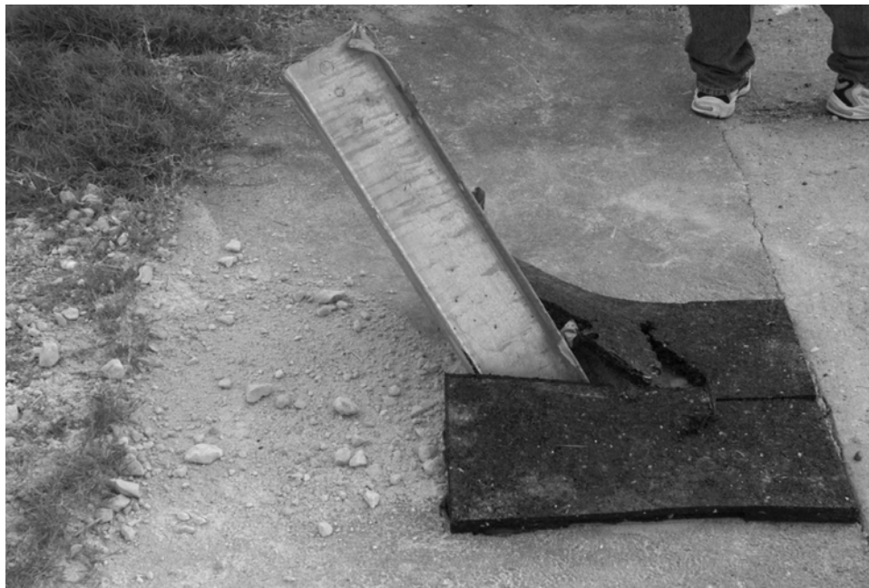
Figure 16. Deformed Steel Post Surrounded by Rubber Mat after Bogie Impact.
