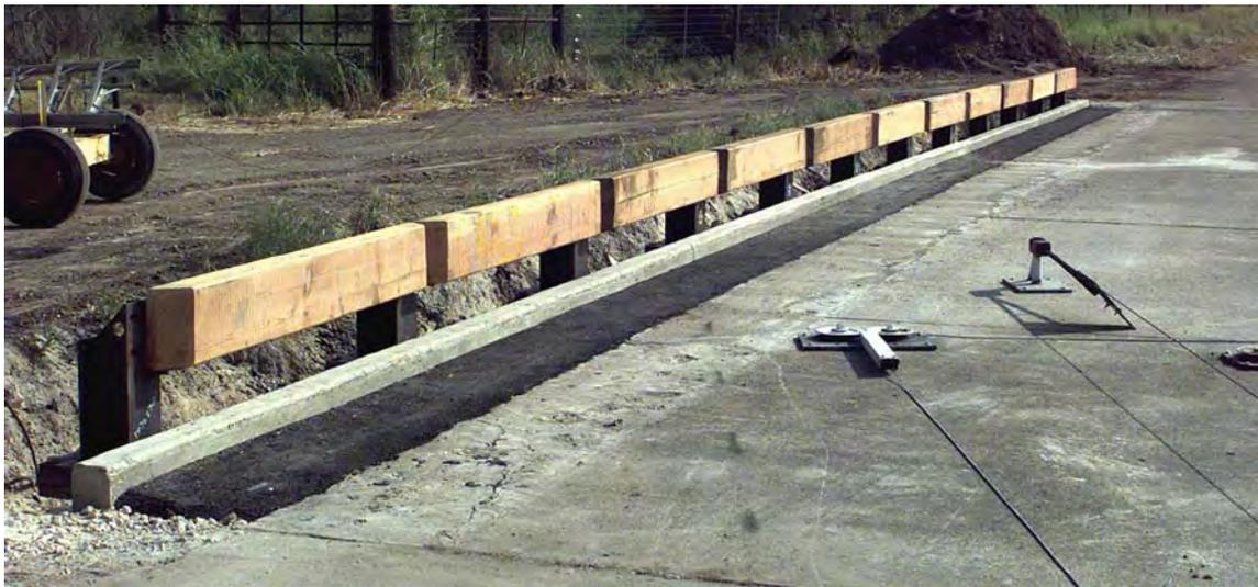
**Figure 14. Glacier Park Removable Timber Guardrail System.**
