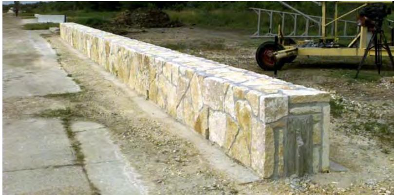
**Figure 8. Rough Stone Masonry Guardwall System.**
