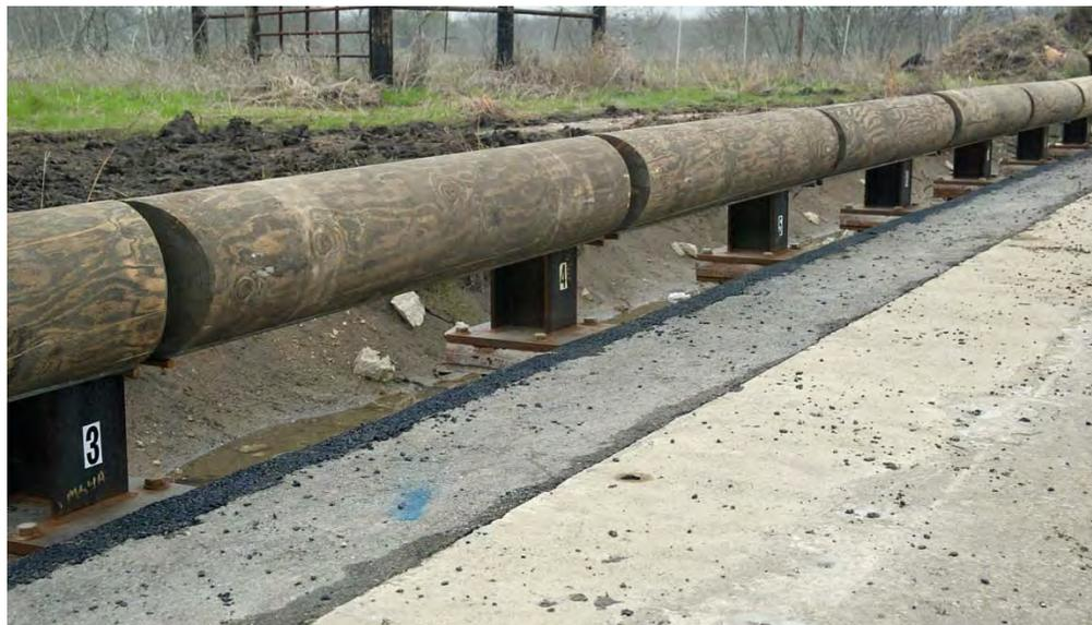
**Figure 15. Glacier Park Round Removable Timber Guardrail System.**
