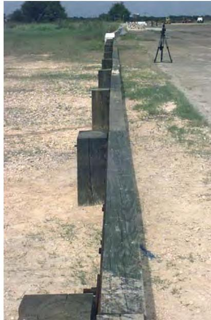
**Figure 11. Type B Steel-Backed Timber Guardrail System.**
