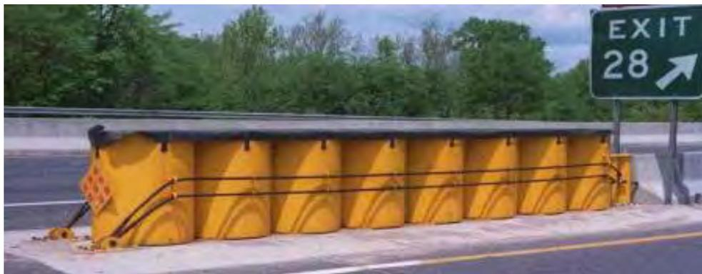
**Figure 30. Narrow Connecticut Impact Attenuator System.**
