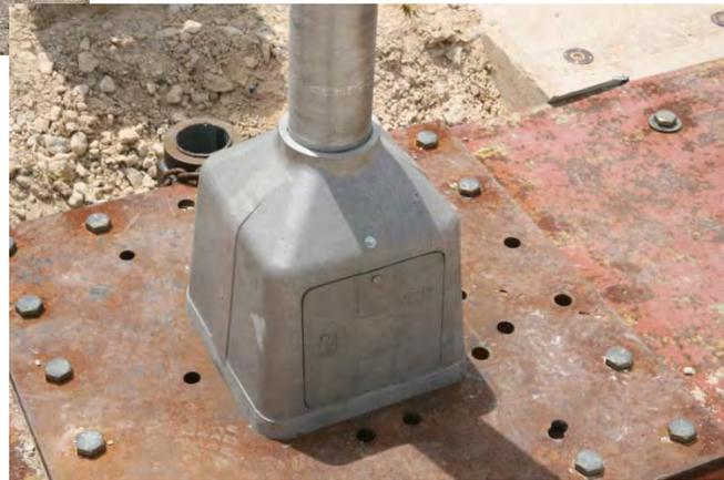
Cast Aluminum Luminaire Support
