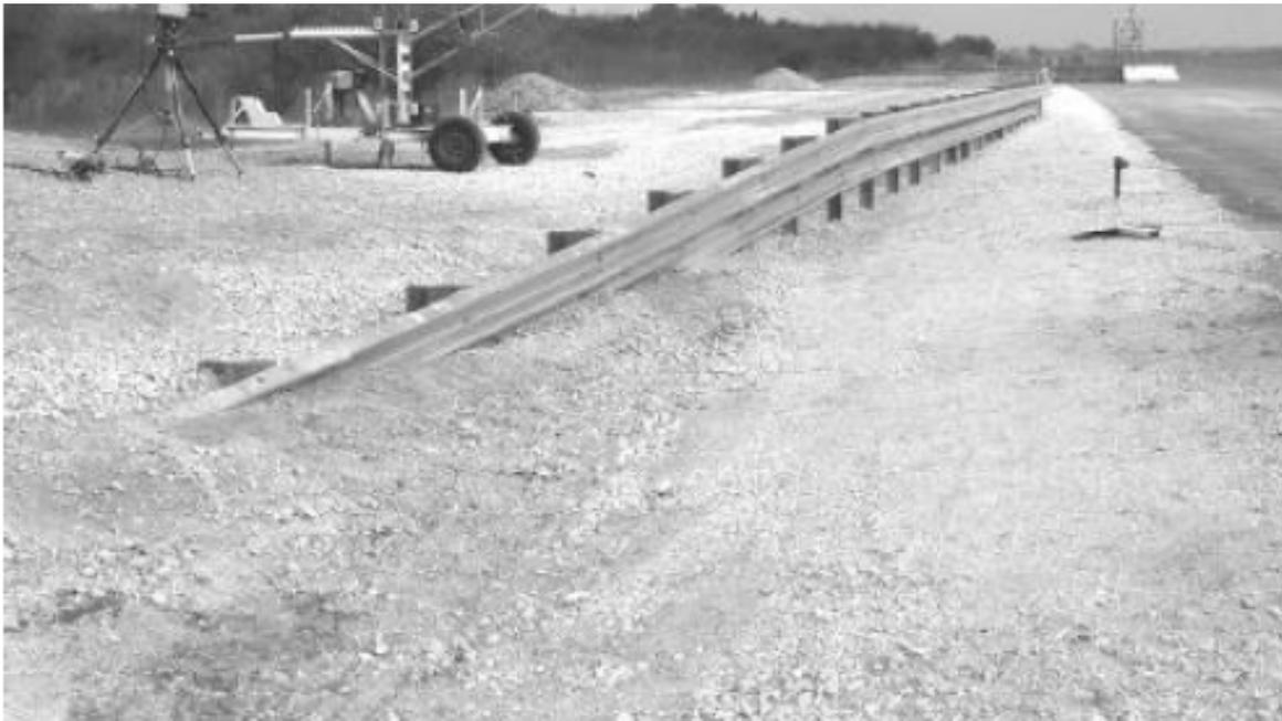
**Figure 24. Buried-in-Backslope Guardrail Terminal.**
