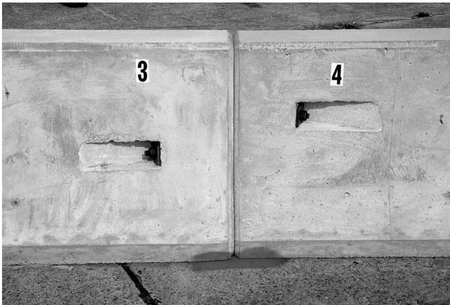
**Figure 21. F-Shape Concrete Safety Barrier with X-Bolt Connection.**
