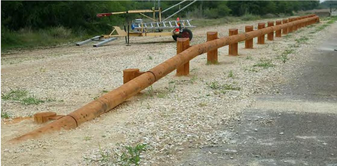
**Figure 12. Round Steel-Backed Timber Guardrail System.**
