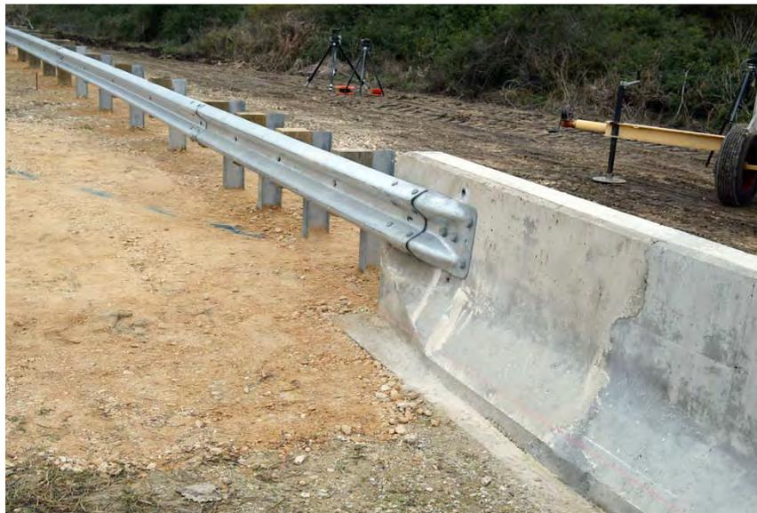
**Figure 23. Texas TL-2 Guardrail-to-Concrete Bridge Rail Transition.**
