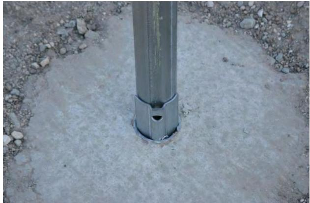
**Figure 33. Photographs of Wedge Anchor Sign Support.**
