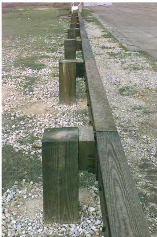
**Figure 9. Type A Steel-Backed Timber Guardrail System.**
