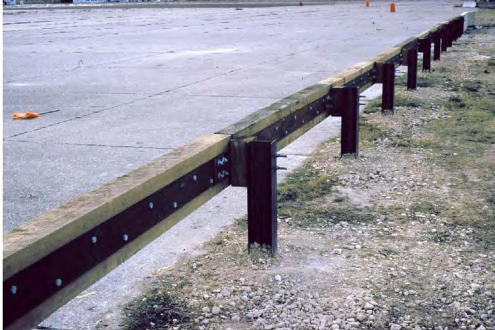
**Figure 10. Merritt Parkway Steel-Backed Timber Guardrail System.**
