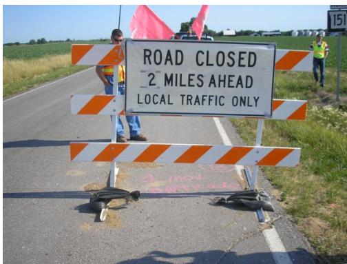
Moveable barricade skid nailed to the pavement to prevent theft
