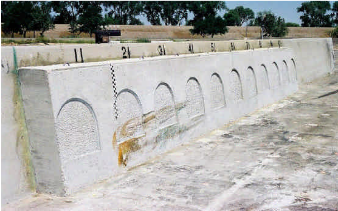
Figure 2-29 Test article after Test 584
