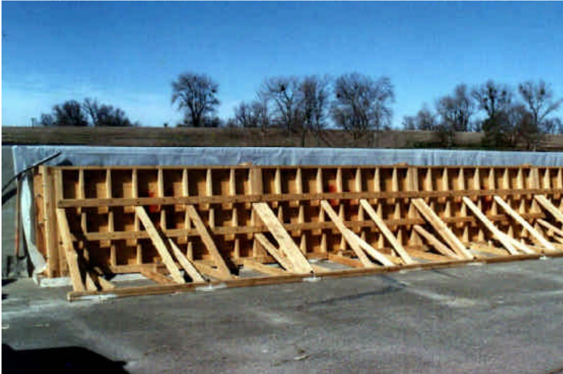
Figure 2-3. Formwork bracing for the 1220 mm high barriers
