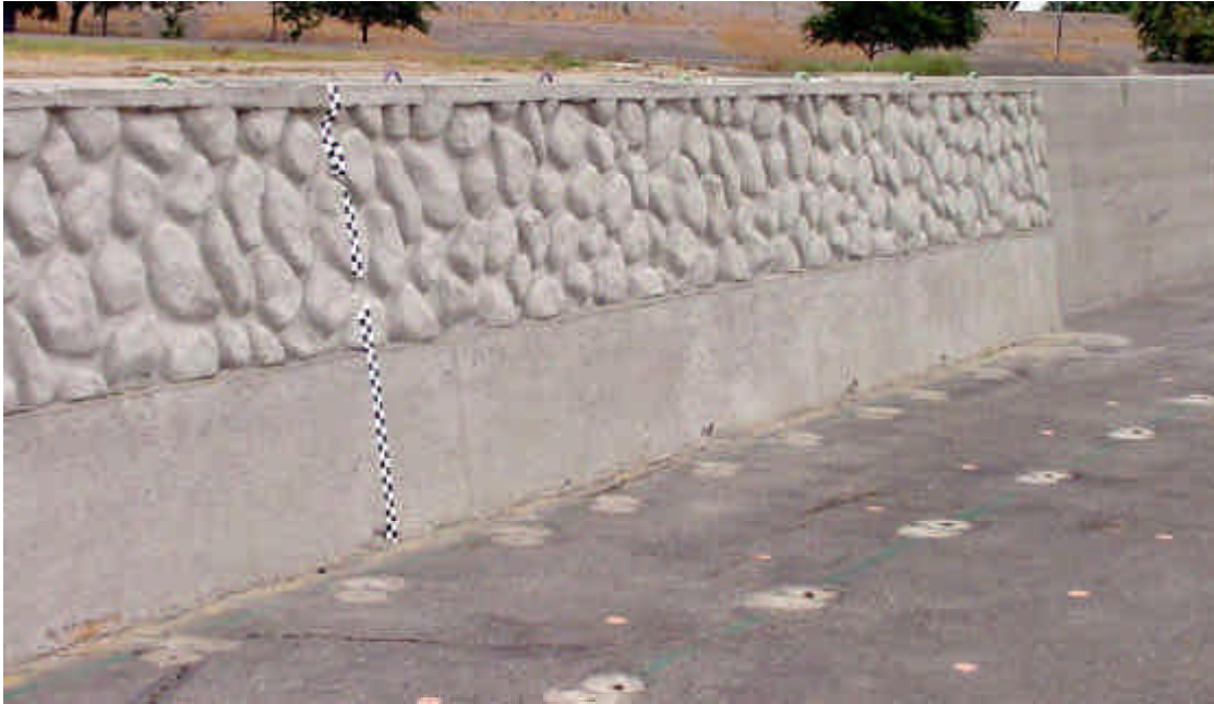
Figure 2-35 Cobble-Reveal test article prior to Test 585 (the cobblestone section of the pattern is the same as that used in Test 581)
