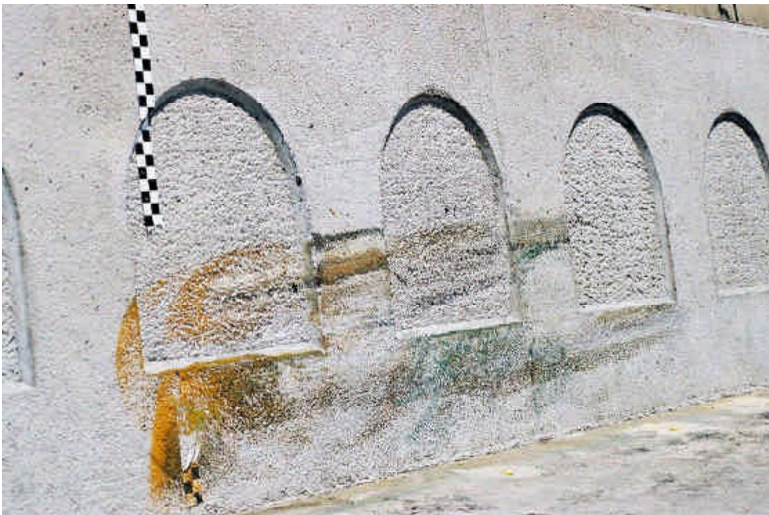
Figure 2-30 Test article after Test 584
