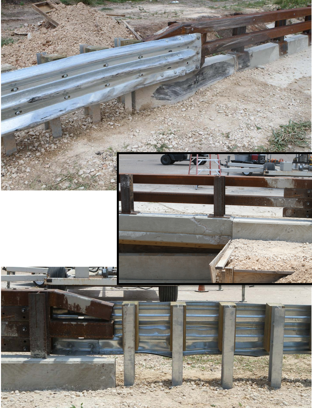
Figure 6.4. TxDOT T131RC Bridge Rail Transition after Test No. 490022-8.
