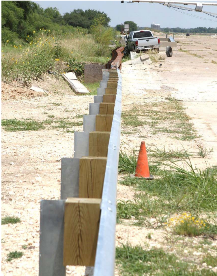
Figure 6.3. Vehicle/TxDOT T131RC Bridge Rail Transition Positions after Test No. 490022-8.
