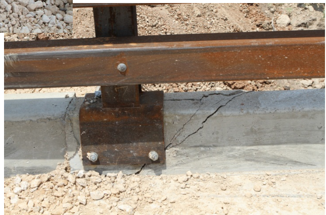
Figure 5.4. TxDOT T131RC Bridge Rail Transition after Test No. 490022-6.
