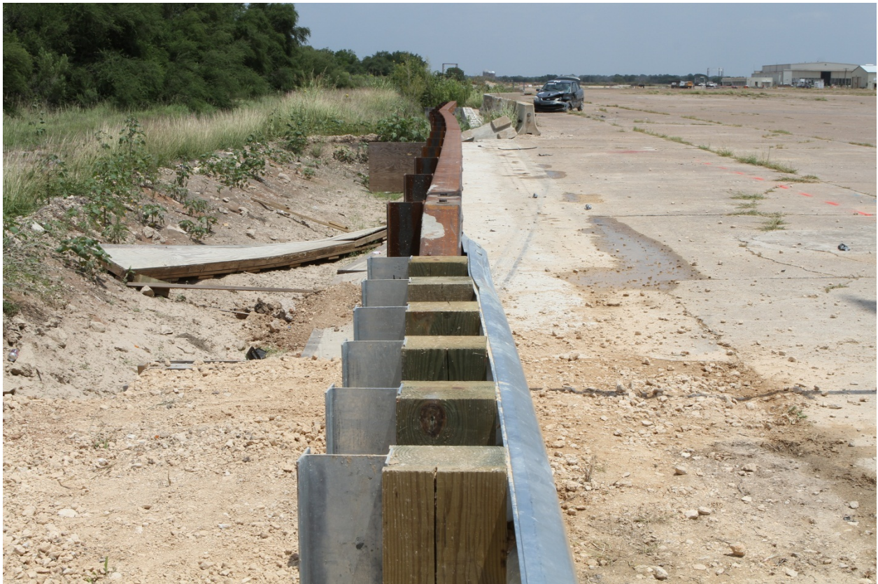
Figure 5.3. Vehicle/TxDOT T131RC Bridge Rail Transition Positions after Test No. 490022-6.
