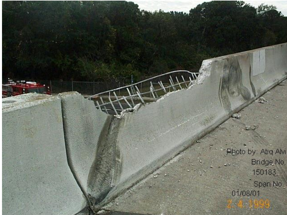
Figure 3. Damage to bridge railing, St. Petersburg, FL...
