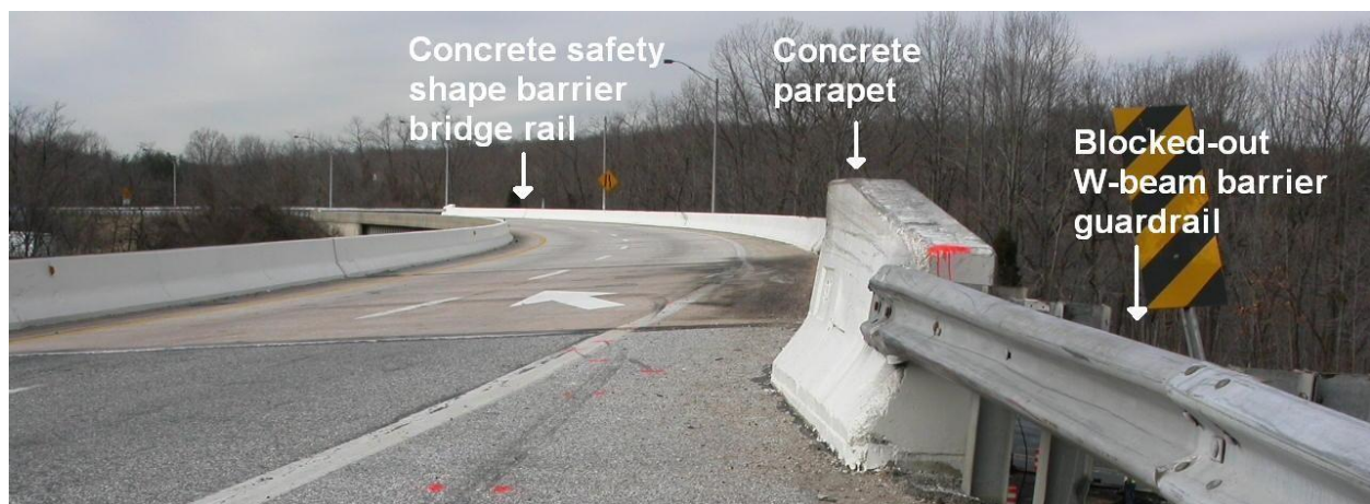
Figure 28. Crash site in Elkridge, MD where a fuel truck penetrated a concrete bridge railing. [NTSB09a]
