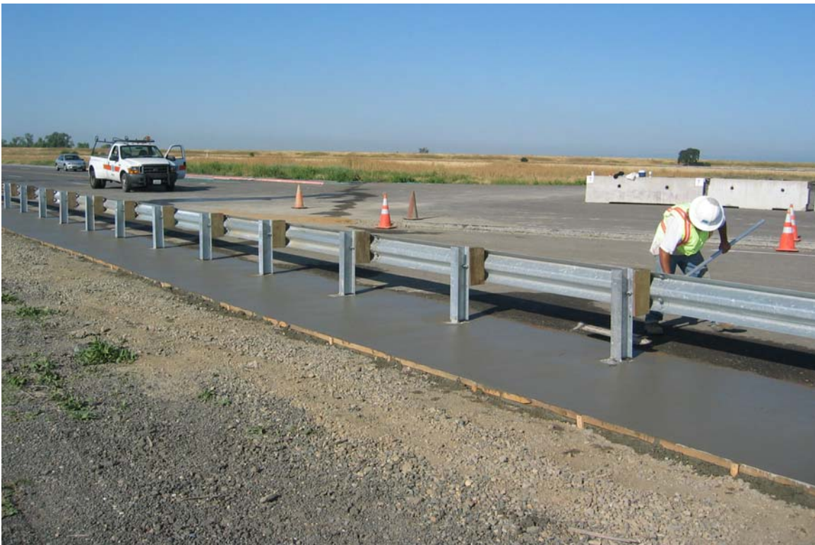
Figure 2-12 – CRMCrete Finishing for Test 658
