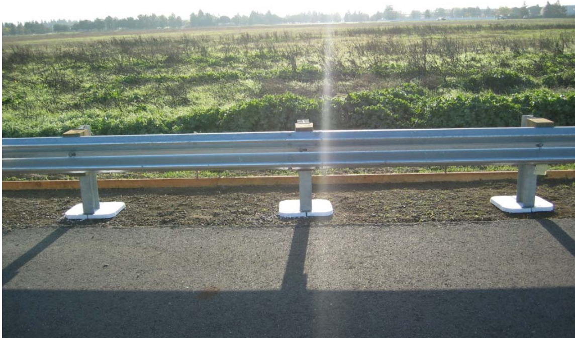
Figure 2-26 – Test 659 Guardrail Prior to CRMCrete Placement
