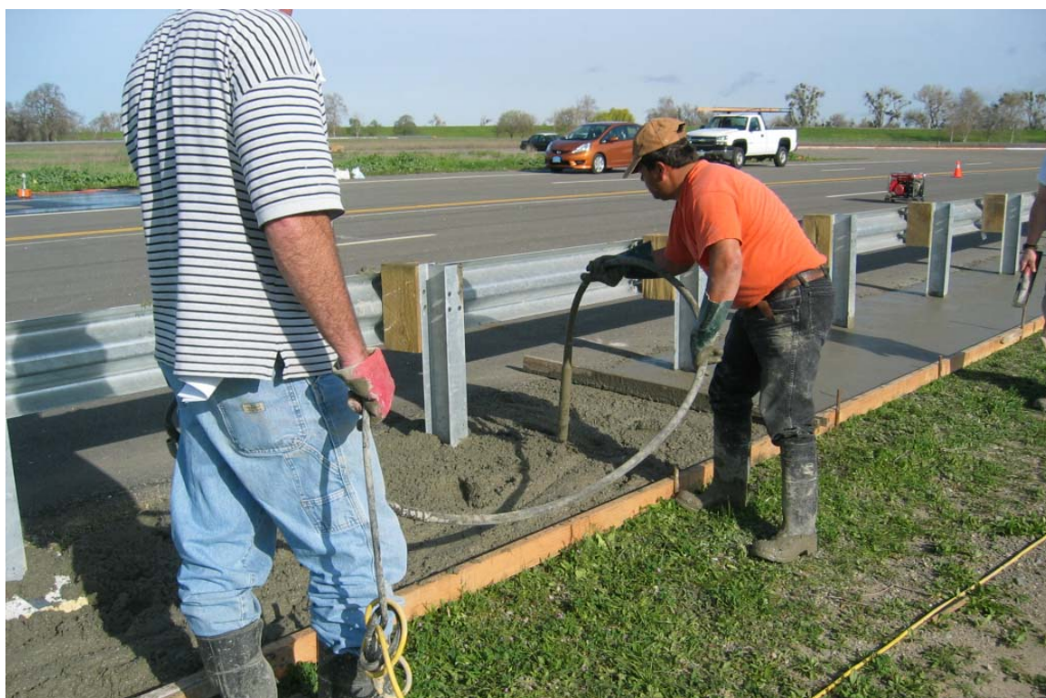
Figure 2-29 – Test 659 Placing of the CRMCrete
