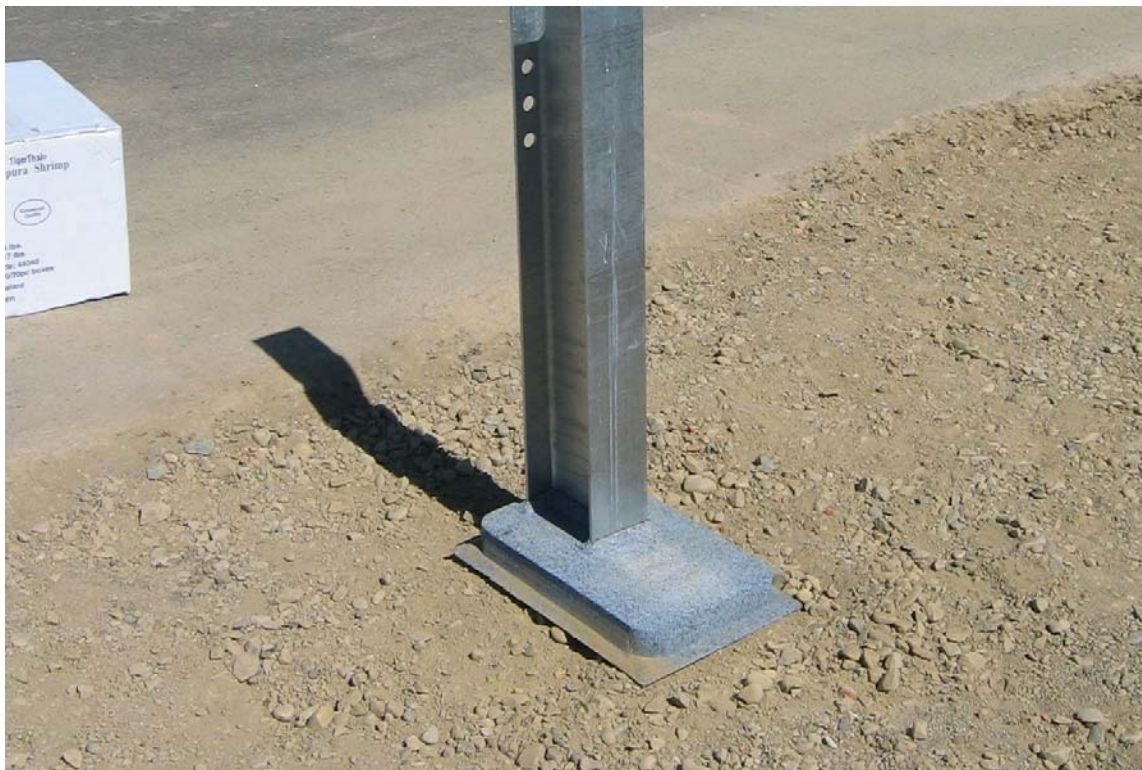
Figure 2-4 – Boot for 2-inch Thick CRMCrete
