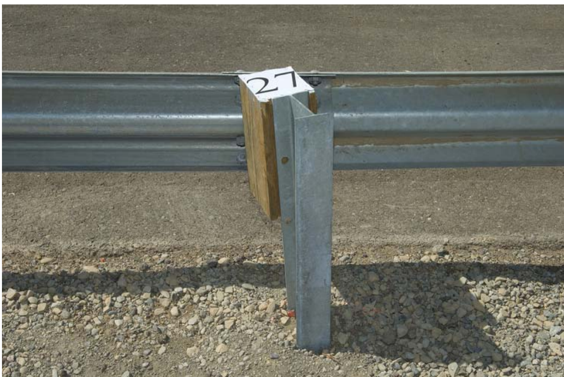
Figure 2-23 – Typical Twisted Post after Test 658
