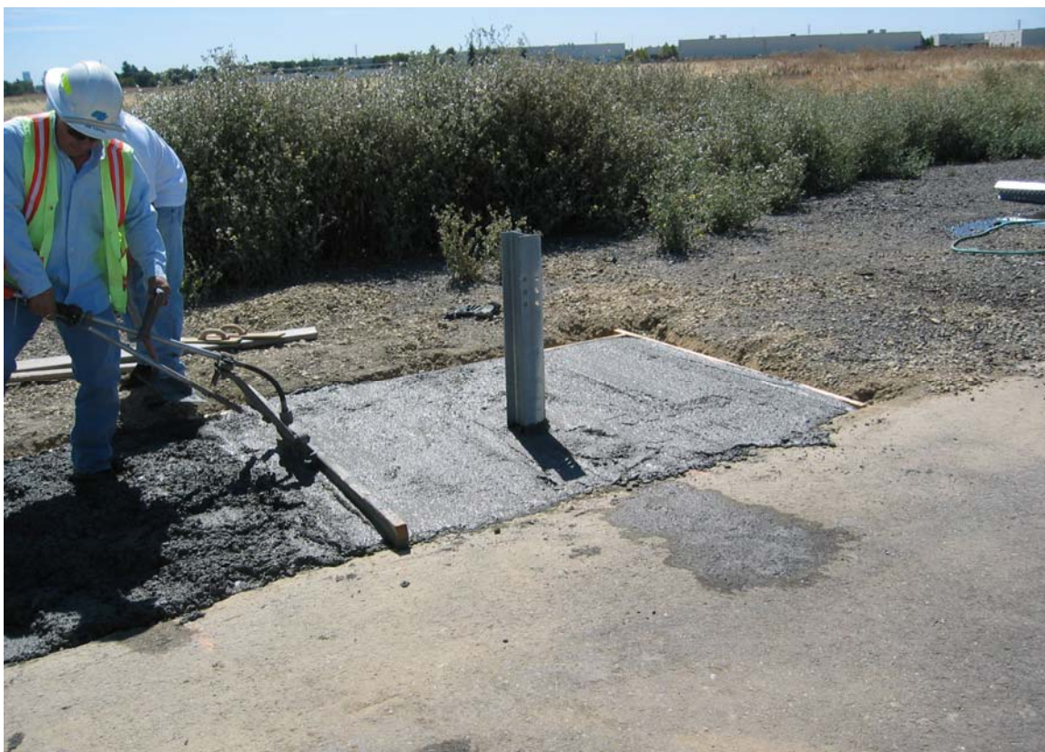
Figure 2-6 – CRMCrete Placement for Bogie Tests
