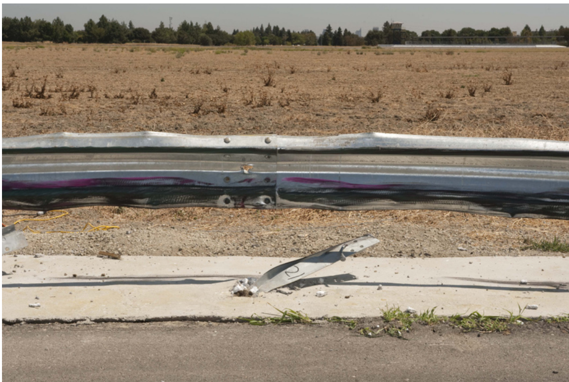
Figure 2-40 – Post 21 (Downstream of Impact Point) after Test 659
