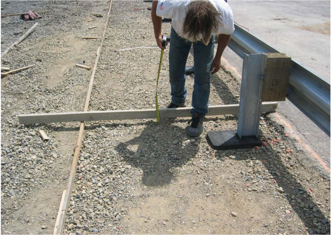
Figure 2-10 – Checking CRMCrete Depth for Test 658
