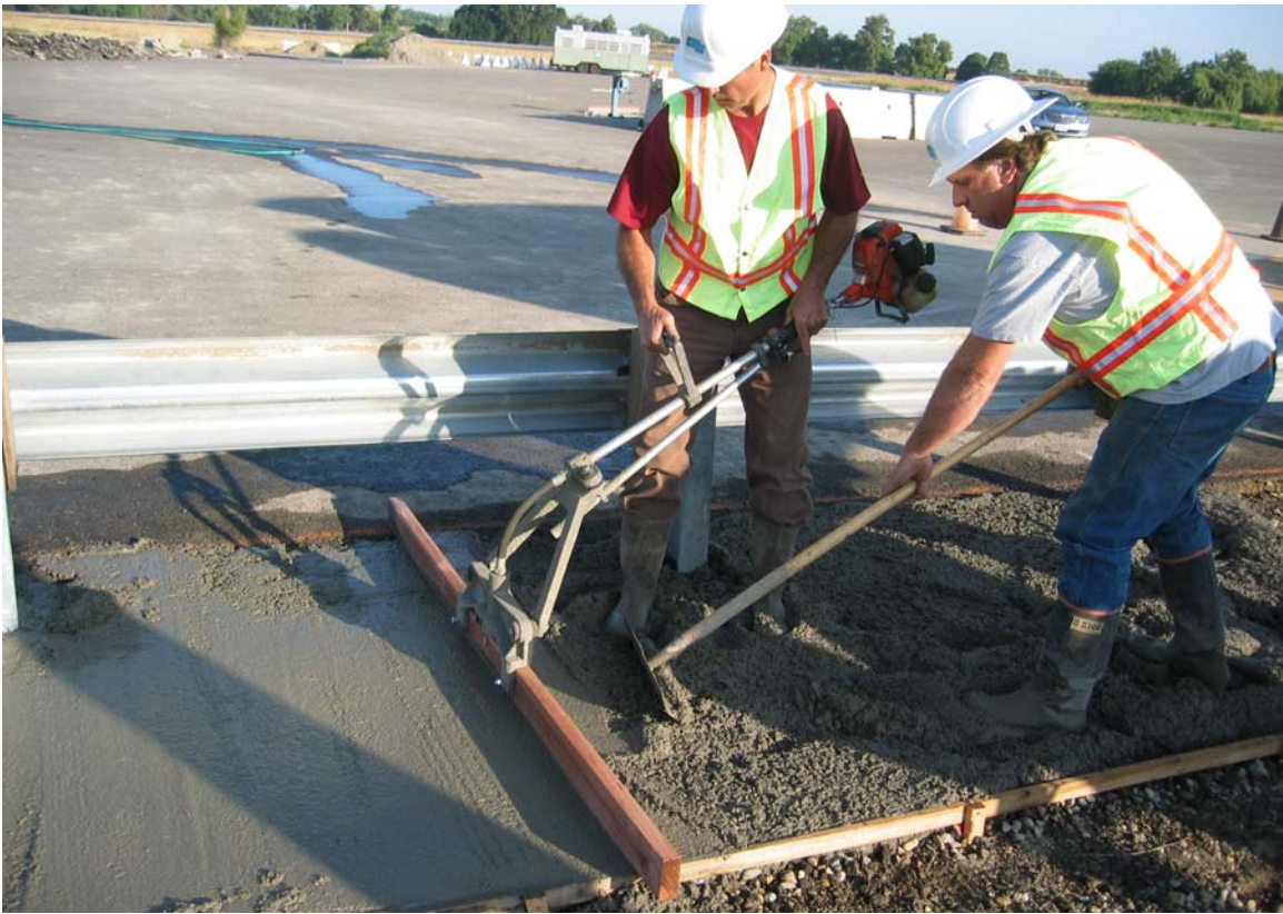
Figure 2-11 – Screeding and Compaction of CRMCrete for Test 658
