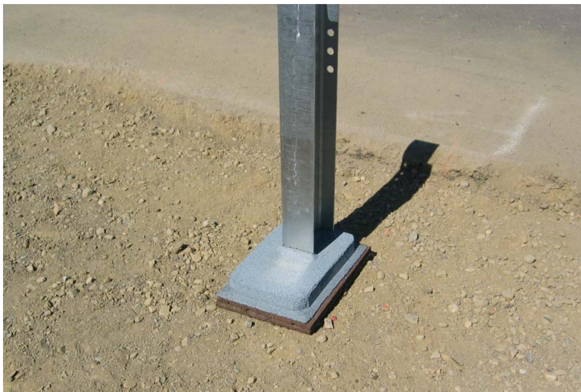
Figure 2-5 – Boot with Spacer for 3.5-inch Thick CRMCrete
