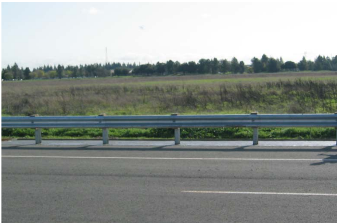
Figure 2-30 – Test 659 Completed Guardrail and CRMCrete Installation
